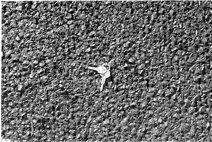
This slide shows OGFC texture.
