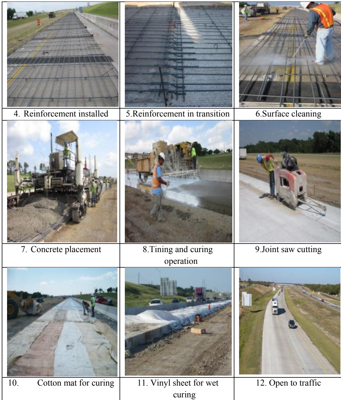
Figure 3.1 Construction sequence of CRCP BCO
