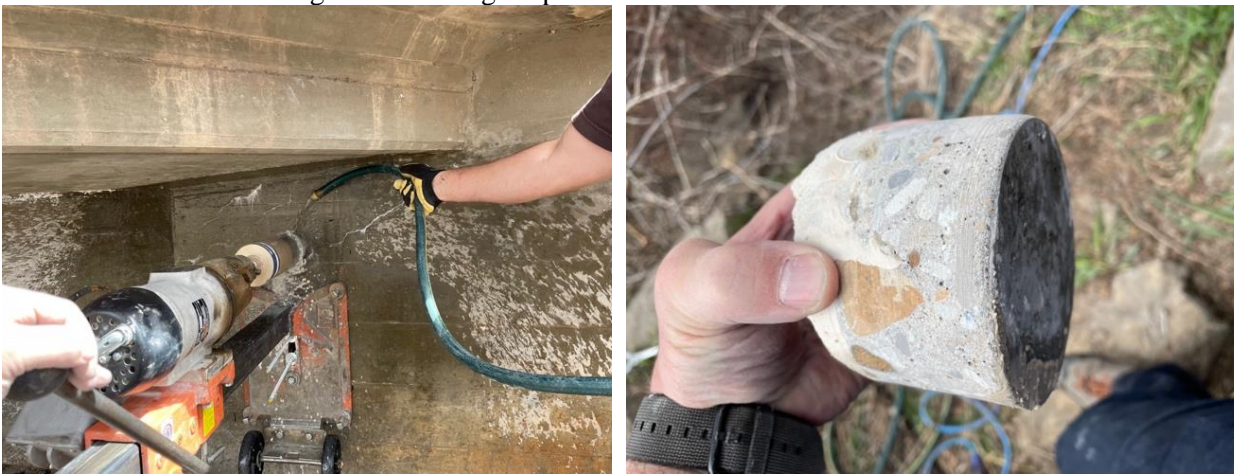
(a) Backwall Coring
