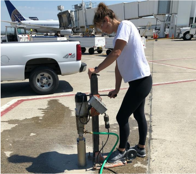
(a) Core Drilling
