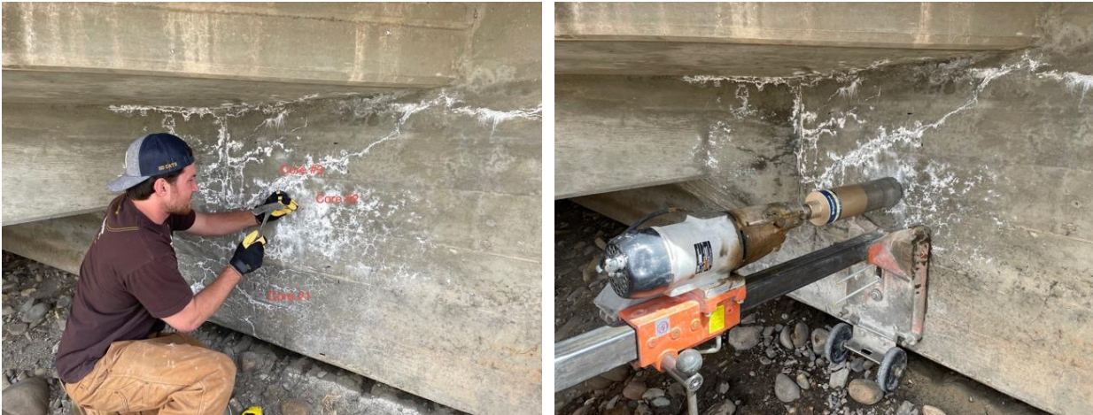
(a) Coring Preparation
