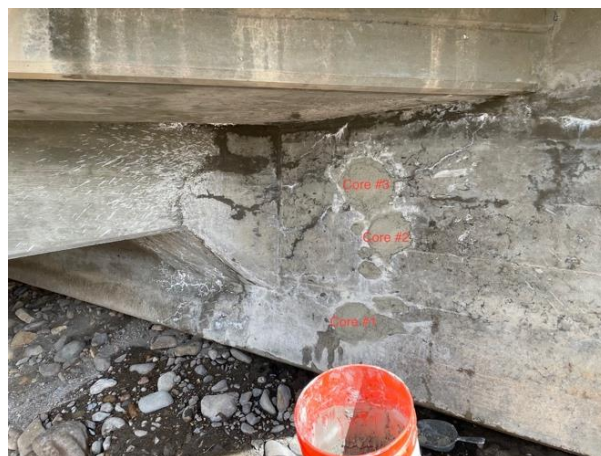
Figure 18: Grouted Core Holes
