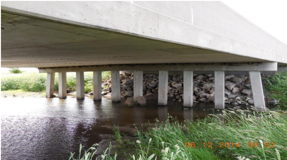
(a) Individually encased piles
