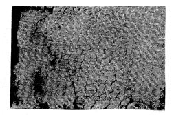
2. Asphalt pavements can deteriorate in a number of ways. Repair methods have generally involved the addition of thickness or the complete removal and replacement of the existing pavement. While both can give satisfactory results, they do not take advantage of the remaining value of the existing paving materials. Cold-mix asphalt recycling is able to recondition the old deteriorated pavement and turn it into a good stabilized base.
