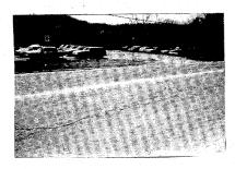
3. This city street exhibits alligator cracking. If left untreated, the cracking will become more severe, reducing the riding quality of the pavement.
