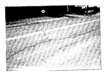
4. A common repair would be to overlay the street with a new layer of asphalt concrete. There is, however, a limit to the number of overlays that can be placed. Too many can cause cross slope, drainage and clearance problems.
