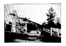
23. The RAP bypasses the dryer, the hot elevator and the screens, entering the weigh hopper directly from a separate conveyor or via an adjacent bin. The RAP should be fed last into the weigh hopper to keep it from sticking to the hopper.
