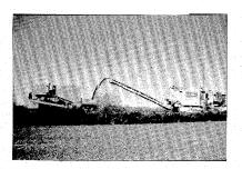
18. Soil stabilization mixing equipment and traveling mixers can be used to add and mix any modifiers. In this view, the RAP is fed from the cold milling machine to a traveling mixing paver.
