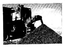
19. Where possible, the removal, crushing, and mixing operations should be coordinated to minimize stockpile size and reduce the problems caused by large piles.
