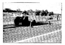
41. The milled roadway surface should be swept with a rotary broom before applying the tack coat. Since the milled surface will be rough with uncoated aggregate surfaces, more liquid asphalt will be needed than for conventional paving.
