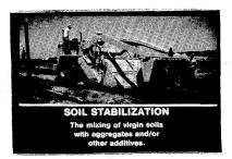
8. Much of the in-place sizing and mixing equipment was developed for soil stabilization work.
