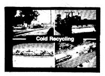
1. In cold-mix asphalt recycling, reclaimed roadway materials are mixed without heat, spread on the roadway and compacted. The reclaimed materials may consist of reclaimed asphalt pavement (RAP), reclaimed aggregate materials (RAM) and untreated foundation materials. New aggregates, modifiers (asphalt and recycling agents) and stabilizers (lime, fly ash and portland cement) can also be added. The mixing can occur either on the roadway or at a central plant.
