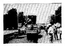
43. Compaction requirements are similar to those for conventional mixes. However, the tendency for excessive dust and fines in recycled mixes may present problems in compacting lifts thicker than 1 1/2 or 2 inches. The density may be 1 to 2 percent less than for a conventional mix with the same compaction effort.
