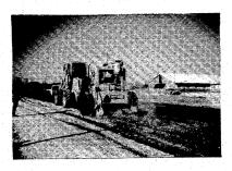
14. The multiple step sequence has the advantage that it uses readily available equipment. However, it has a number of disadvantages. It cannot be used on projects where only partial depth removal is planned. There is usually some mixing between the RAP and the base and some oversized RAP may remain. Production rates are slow and there may be problems with equipment coordination and traffic control.
