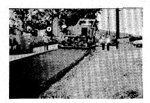
34. Conventional equipment can be used to lay and compact cold recycled mixes.
