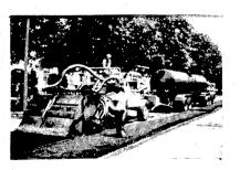
28. Mixing operations are often performed with single and multiple transverse shaft rotary (flat type) mixers. The modifier can be applied either to the windrow by an asphalt distributor or by a spray-bar in the cutting chamber.
