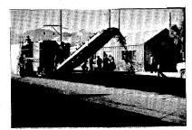
16. Cold milling machines have rotating drums lined with cutting teeth to grind the old pavement. They provide accurate depth and profile control, the ability to pulverize and size in a single pass and high productivity. However, they require trained personnel, have higher operating costs and may generate excess fines.
