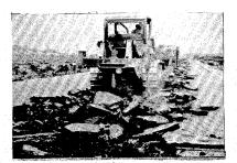
6. One method of removing and sizing the RAP is to break up the pavement using rippers, grid rollers, earthmoving equipment, or scarifiers. The RAP is then loaded into trucks and hauled to a hot-mix plant where it is crushed.
