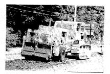
32. A number of options for removing and sizing RAP are associated with central plant cold-mix asphalt recycling. These vary based on the amount of sizing done on-site. The method chosen will probably be determined by equipment availability and the acceptability of extended road closures.
