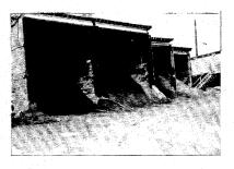
16. RAP has a tendency to absorb moisture because of its higher content of fine particles. Since the heat required to evaporate this moisture comes from the super-heated virgin aggregate, higher moisture contents will result in lower production rates or in less RAP being used. Protective coverings can be effective. Drainage should be provided to prevent water from accumulating under the stockpile.
