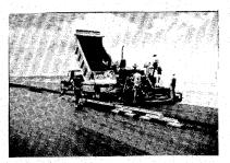
42. Paver characteristics, lift thicknesses and mix properties will influence the uniformity, laydown, compaction, and rideability of the mat. The extra fines generated by cold milling can cause the mix to be stiff, resulting in pulling of the mat and lower mat density.
