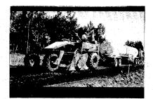
13. Mixing of the RAP with modifiers and stabilizers can be done by motor grader or traveling mixers.
