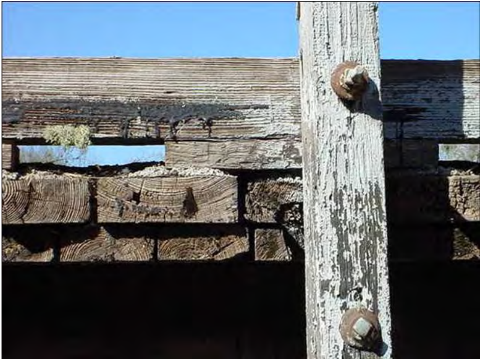
Coatings on wood posts or timber piles
