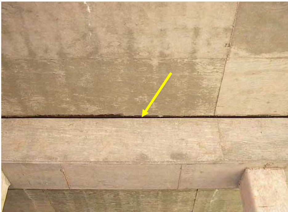
Roofing felt or fiberboard bearing material
