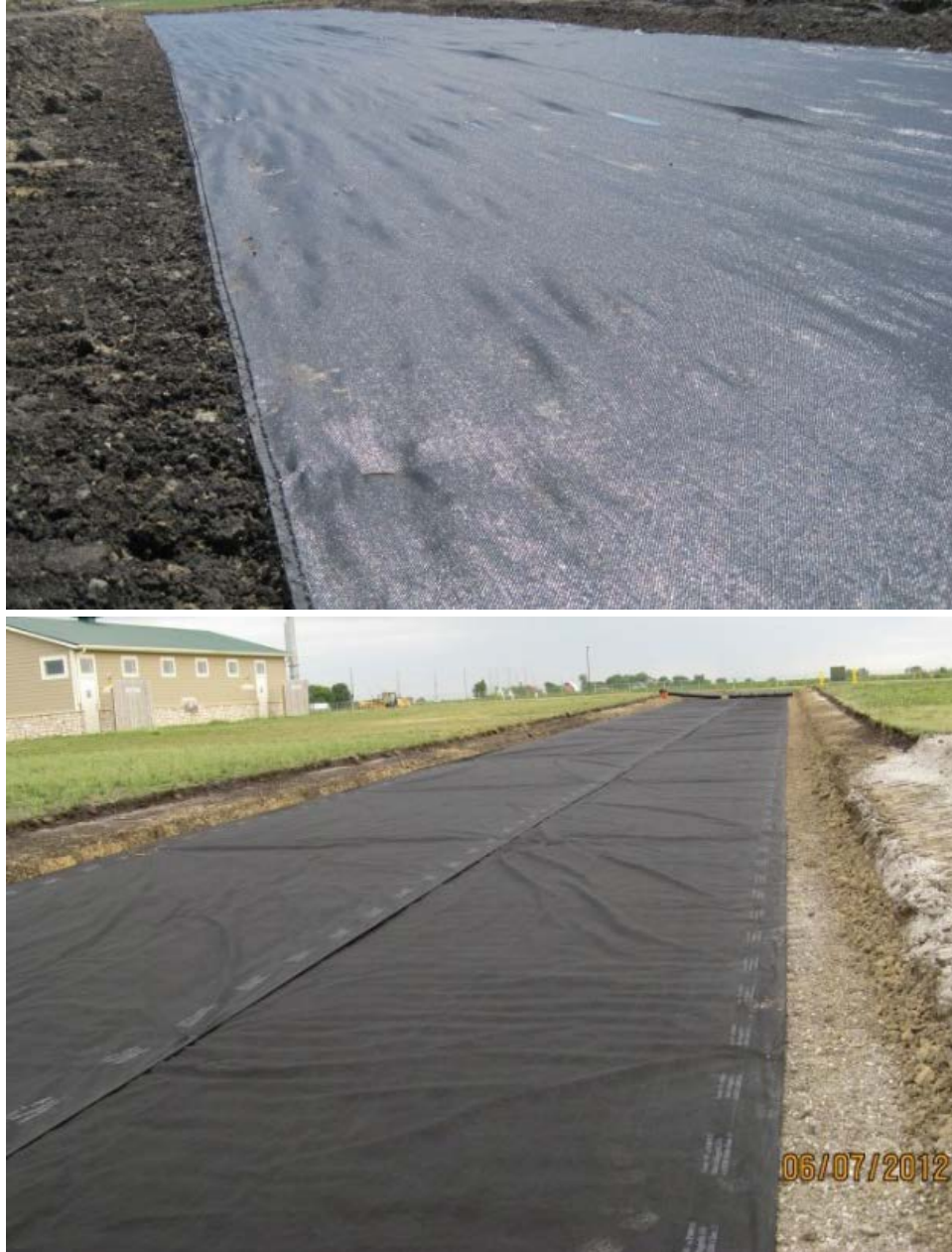
Figure 4. Woven geotextile (left) and non-woven geotextile (right) placed at subgrade/aggregate layer interface
