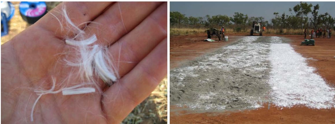
Figure 7. Polypropylene fibers (left) and distribution of fibers and mixing with cement (right) (Newman and White 2008)
