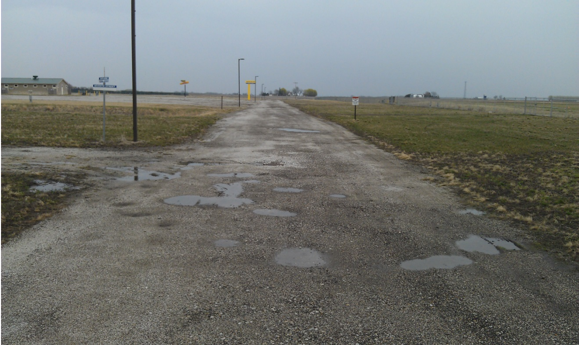
Figure 37. Conditions of South Ave. in April 2012
