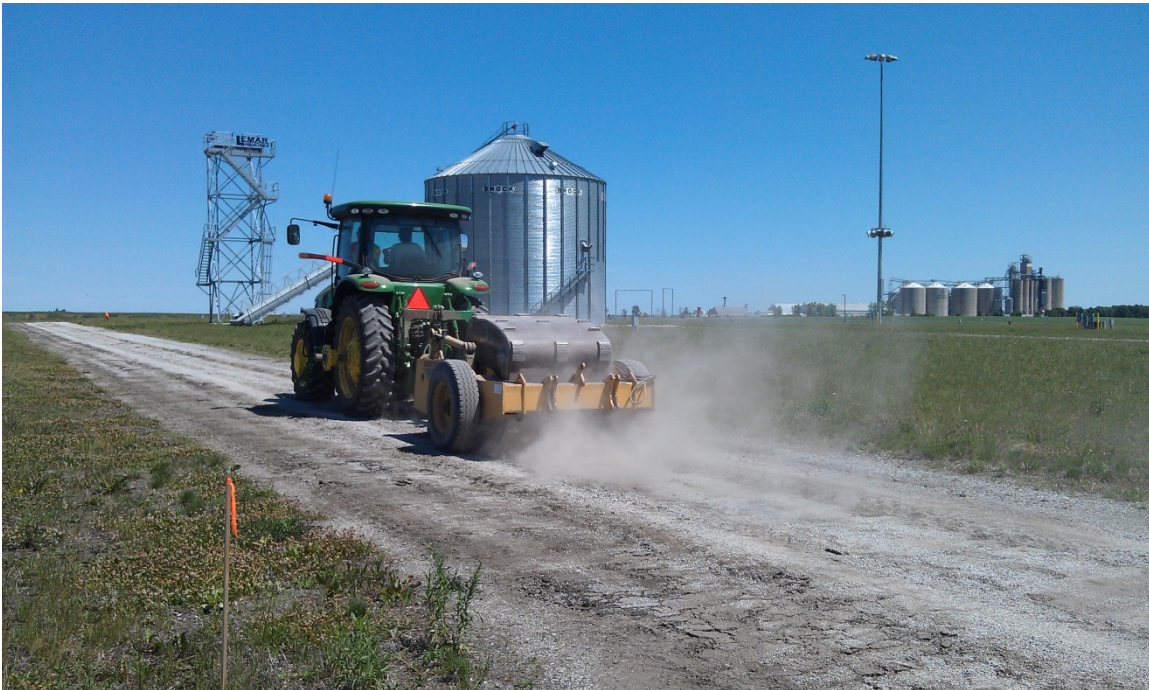
Figure 8. High energy impact compaction (HEIC) roller manufactured by Impact Roller Technology in Plattsmouth, Nebraska
