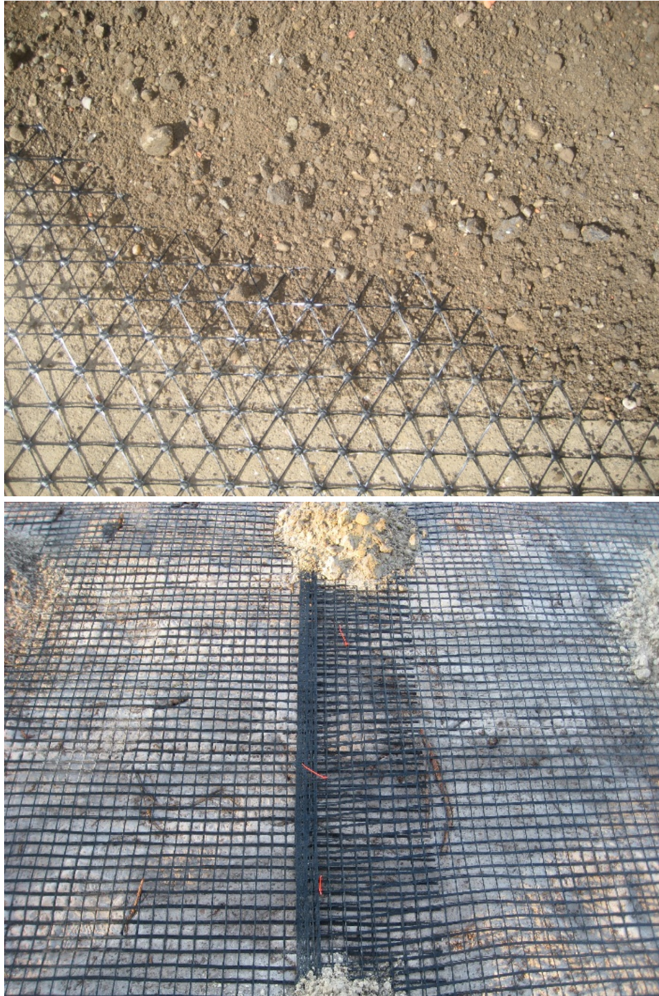
Figure 5. Triaxial (left) and biaxial (right) polymer geogrids placed on the subgrade
