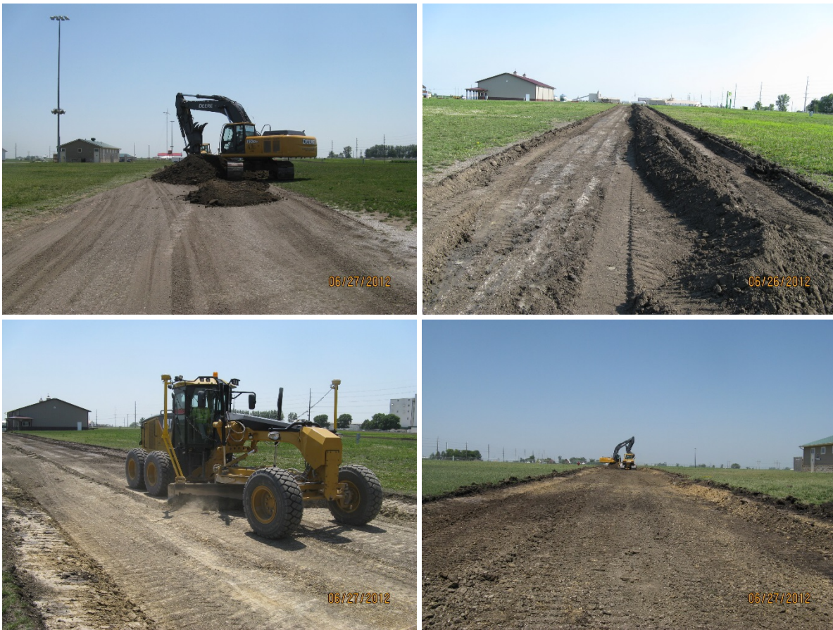
Figure 80. Removal of existing granular subbase on 3rd St.
