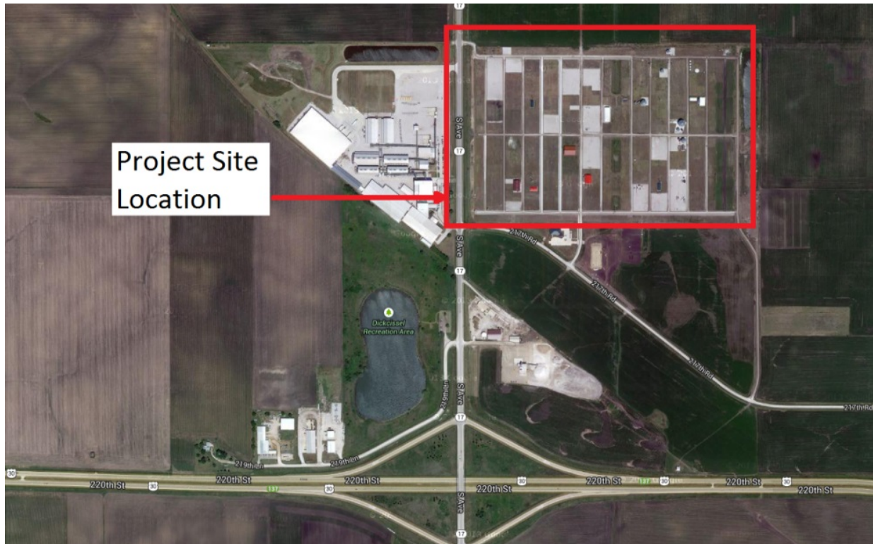
Figure 34. Aerial imagery of CIE site in Boone County, IA
