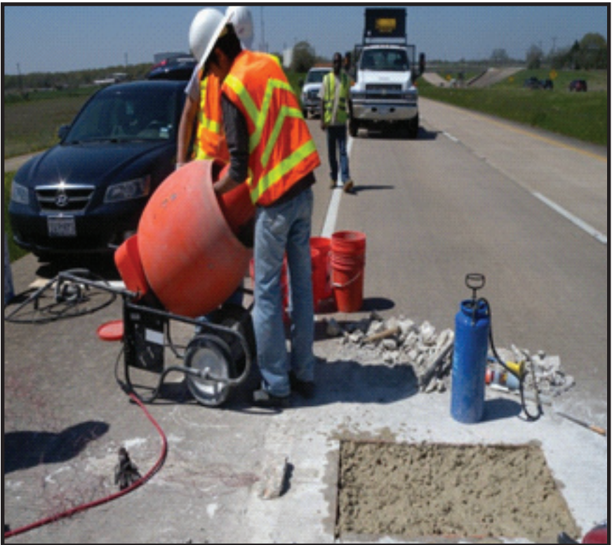
Figure 11. Mixing of prepared repair materials at the job site
