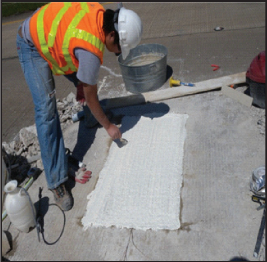
Figure 12. Application of sufficient curing compound
