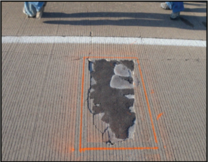
Figure 7. Boundary of PDR straight and clearly marked
