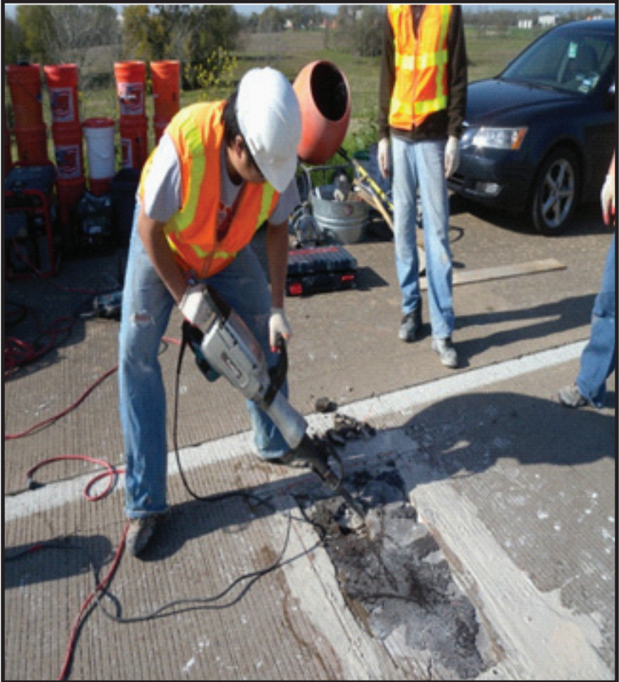
Figure 9. Removing concrete using a jackhammer
