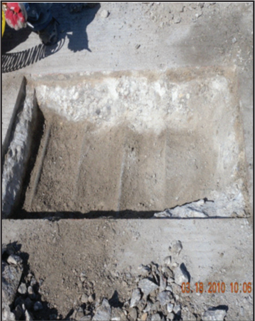
Figure 10. Large amount of fine materials at the bottom of the PDD
