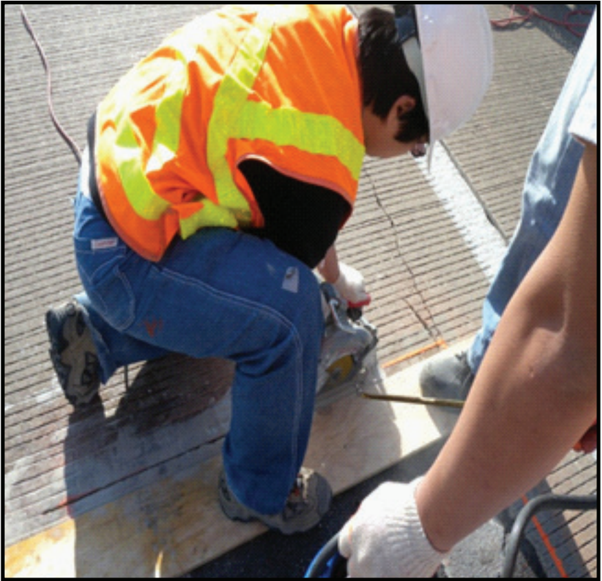
Figure 8. Saw cut operation
