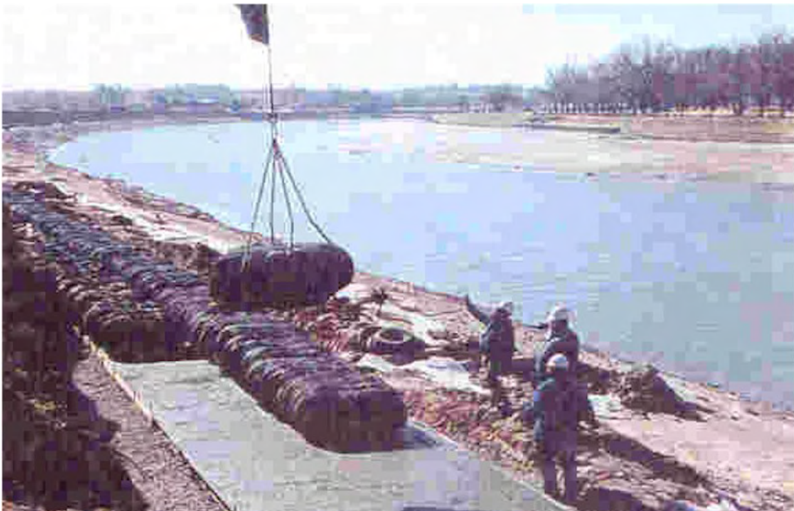
Figure 5.8 Placement of One-Ton Tire Bales onto Concrete Base (NMED 1999)
