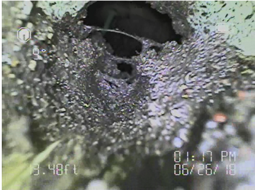
Figure 3.31. Entrance of south access port under west approach of Bridge 5622.50061.
