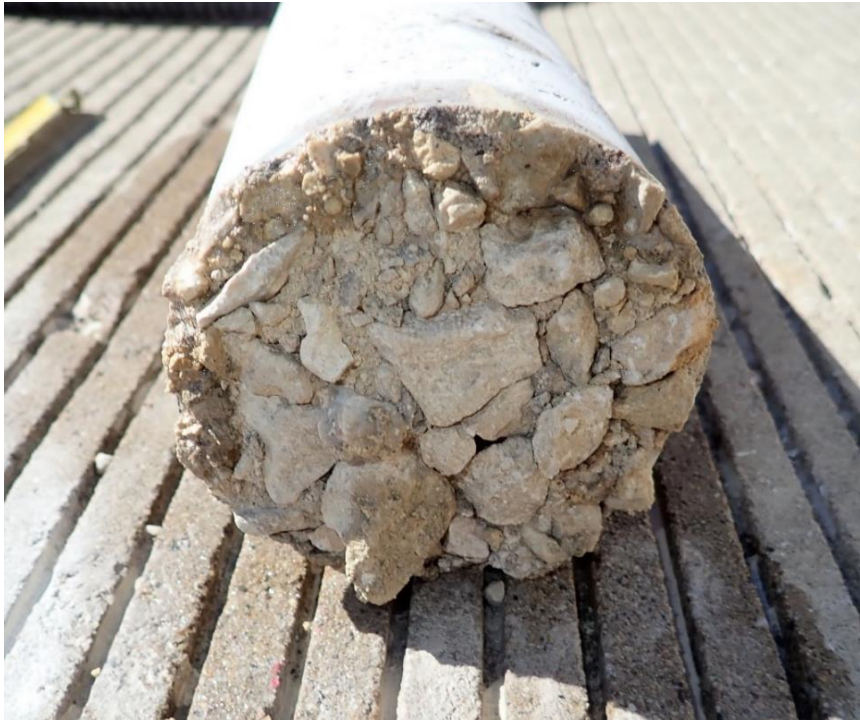
Figure 3.37. Bottom of Core 1 of Bridge 5624.20061, showing original contact with the base.
