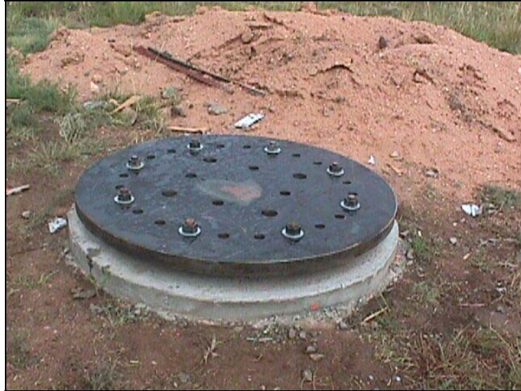
Figure 3.5 Foundation with Steel Plate
