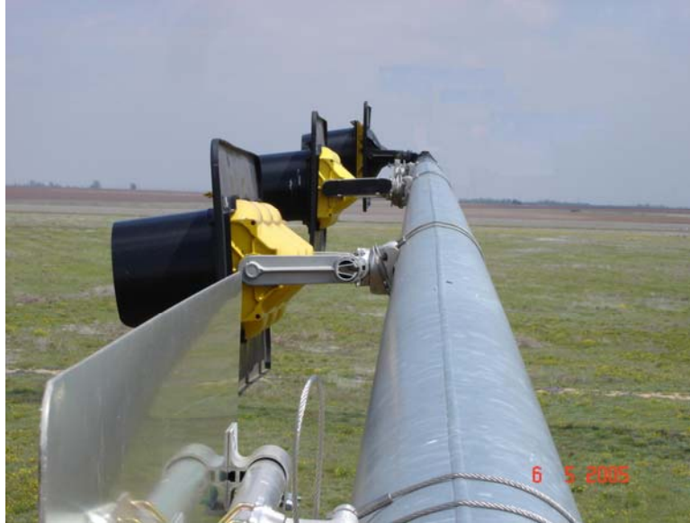
Figure 7.1. Traffic Signal Configuration Susceptible to Vortex Shedding
