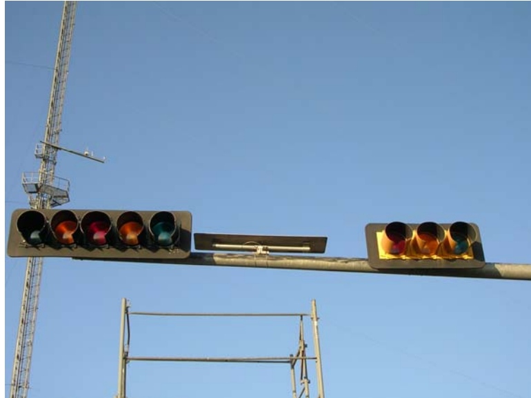
Figure E. 23 Mast arm with damping plate
