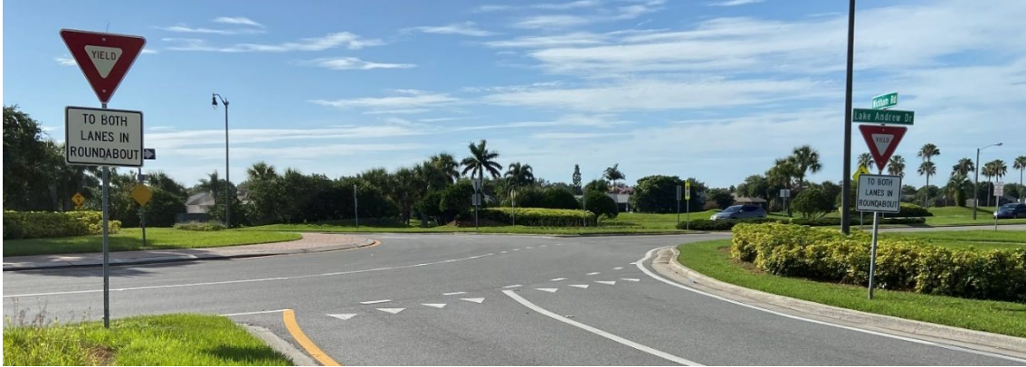
Figure 80. Photo. Melbourne entrance line and parallel yield line.
