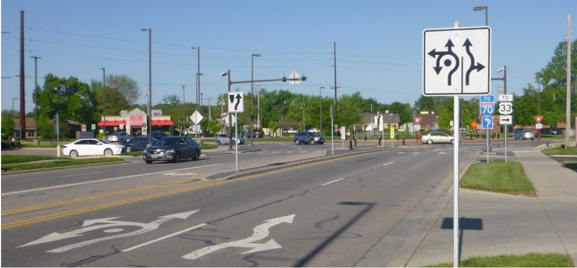
Figure 82. Photo. Hilliard side-mounted lane-use sign and two sets of fishhook markings.
