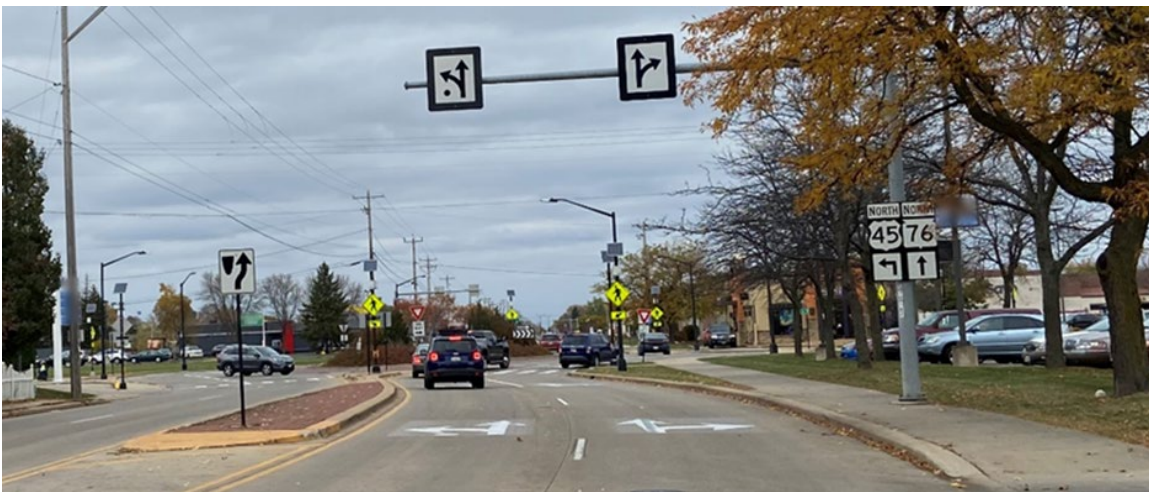
Figure 82. Photo. Hilliard side-mounted lane-use sign and two sets of fishhook markings.
