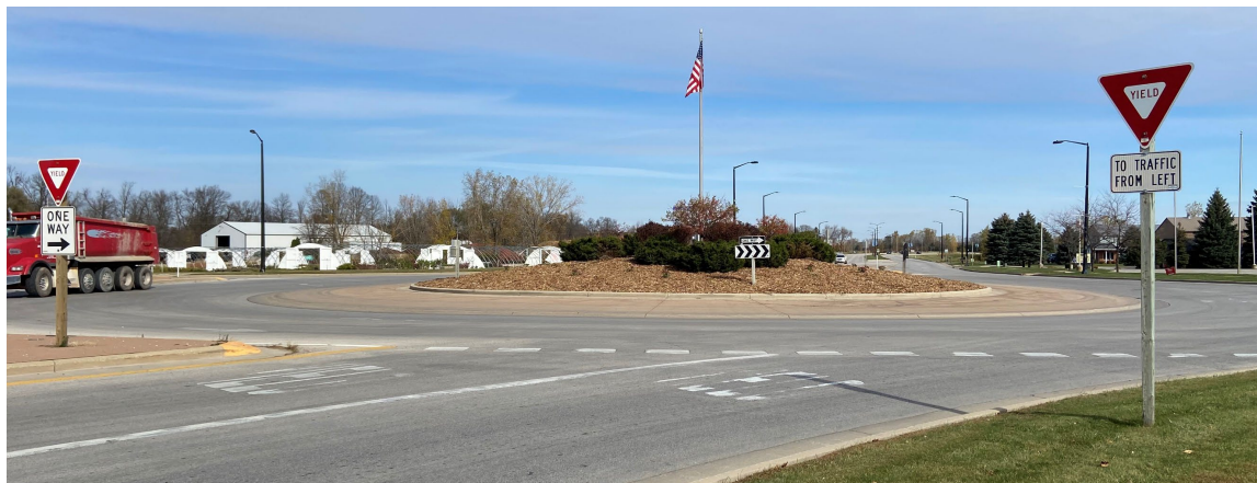
Figure 76. Photo. De Pere—Yield signs with a one-way sign and a ‘TO TRAFFIC FROM LEFT’ supplemental plaque.
