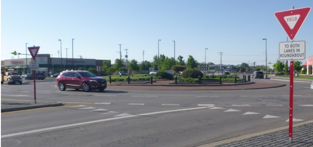
Figure 77. Photo. Hilliard yield signs with ‘TO BOTH LANES IN ROUNDABOUT’ supplemental plaques.
