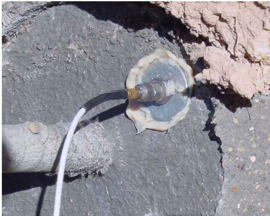
Figure 3 Accelerometer Attached to Washer on the Grout
