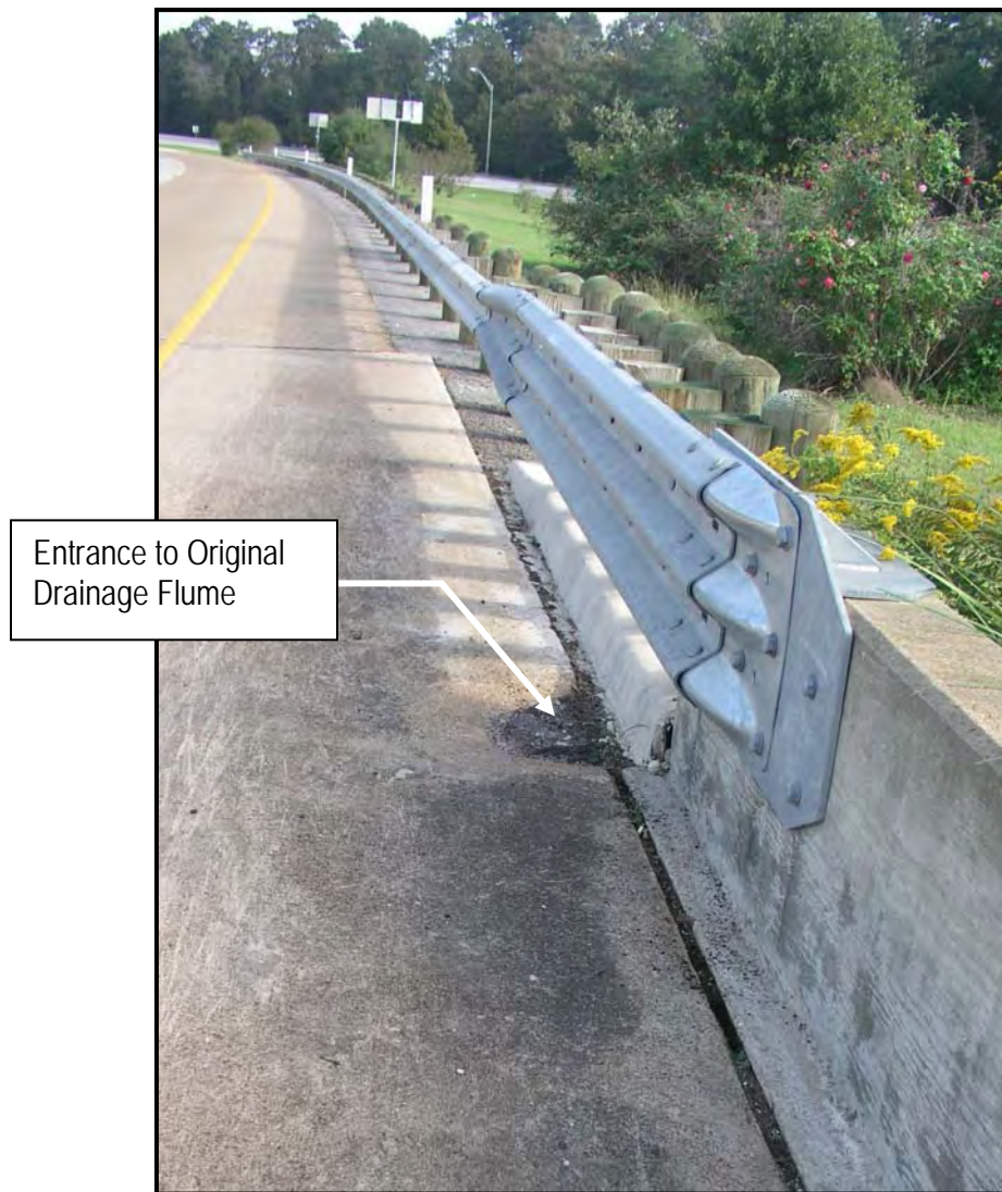
Figure 5.8 Entrance to Original Drainage Flume Blocked by the Installation of the Monocurb in the New Thrie Beam Guardrail System
