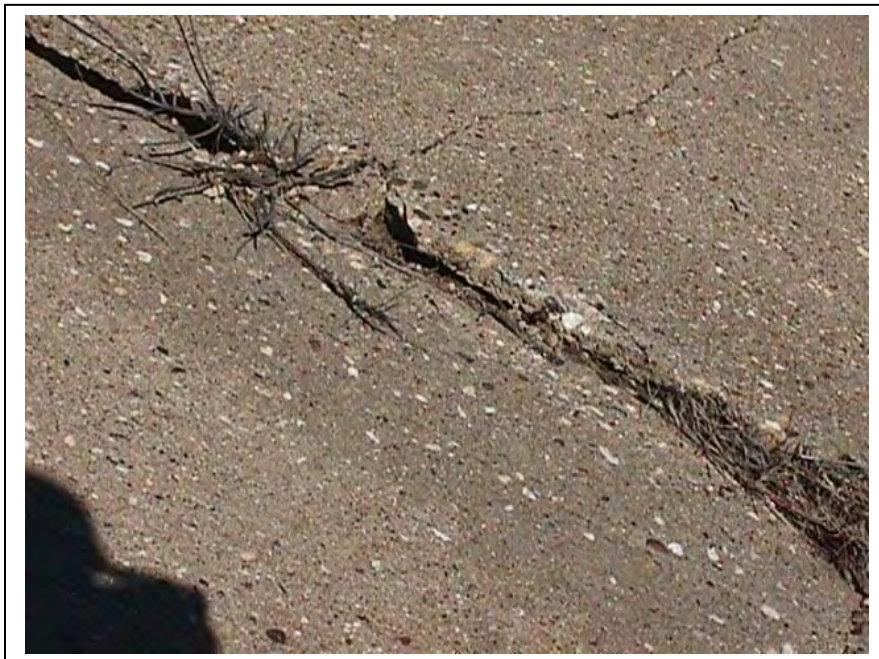
Figure 4.3 Damaged Joint in Riprap Slab
