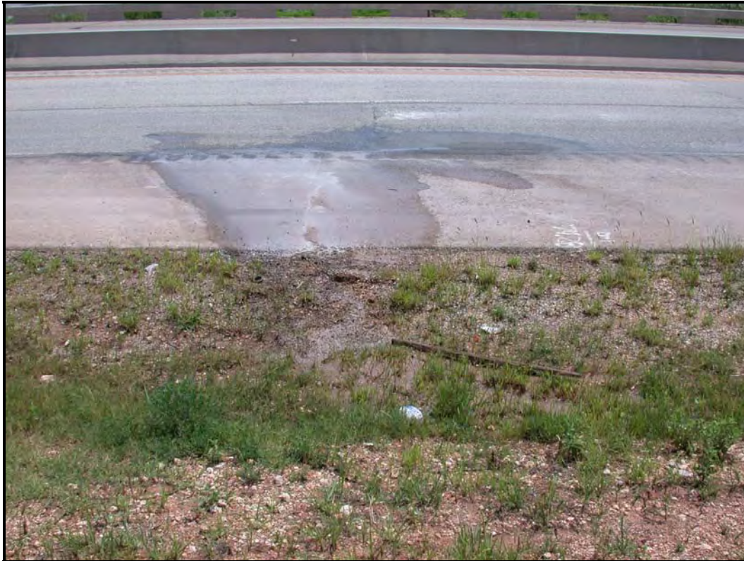
Figure 5.3 Water Seepage at the US-83 Overpass Bridge Departure over Antilley Road in Abilene District
