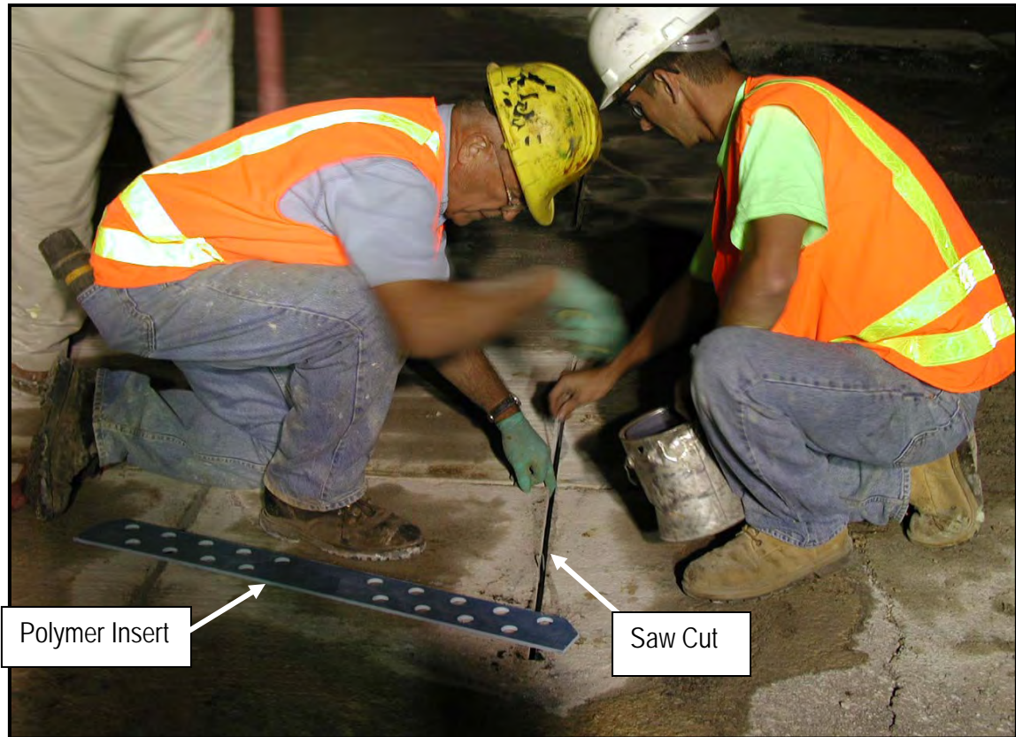
Figure 5.21 Sawcut Prepared to Receive Polymer Insert
