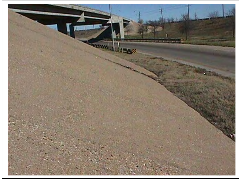
Figure 4.4 Differential Settlement of Riprap Slab (Side View)
