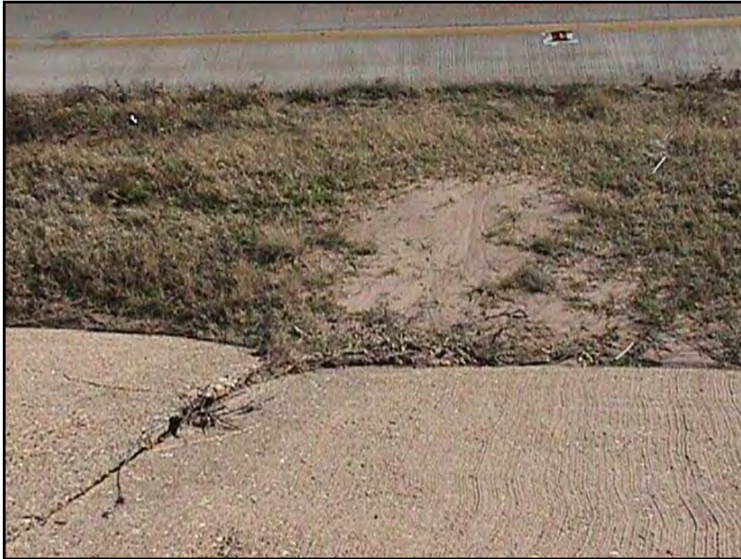
Figure 5.2 Signs of Embankment Fill Erosion at IH-27 Overpass over 4 th Street in Lubbock District
