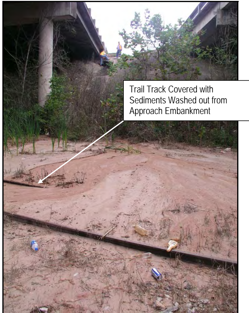
Figure 5.1 Extensive Erosion at Business 69 Overpass over Southern Pacific Railroad in Lufkin District
