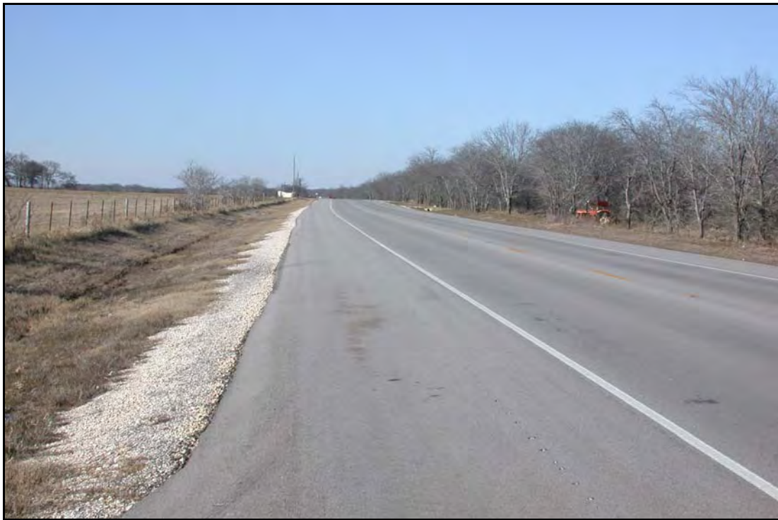
FIG. 6.4 FM 933 Road Rehabilitation, Waco District (see Waco District Profile, Photo 16)
