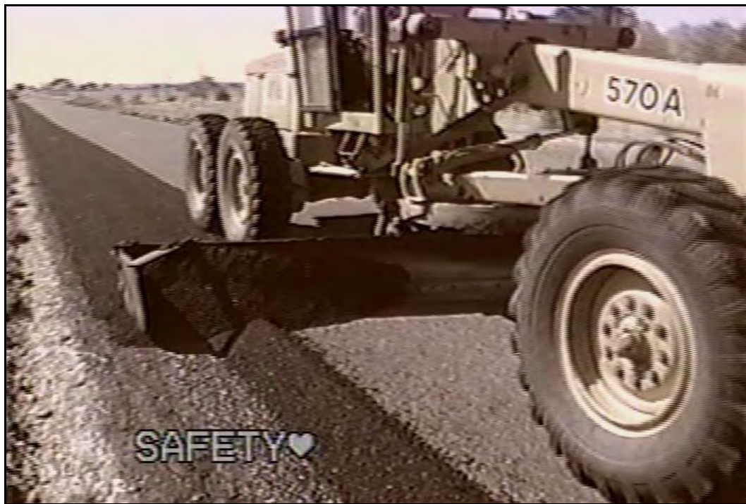
FIG. 7.7 Motor Grader Blade Shoe for Reshaping Shoulders, Waco District
