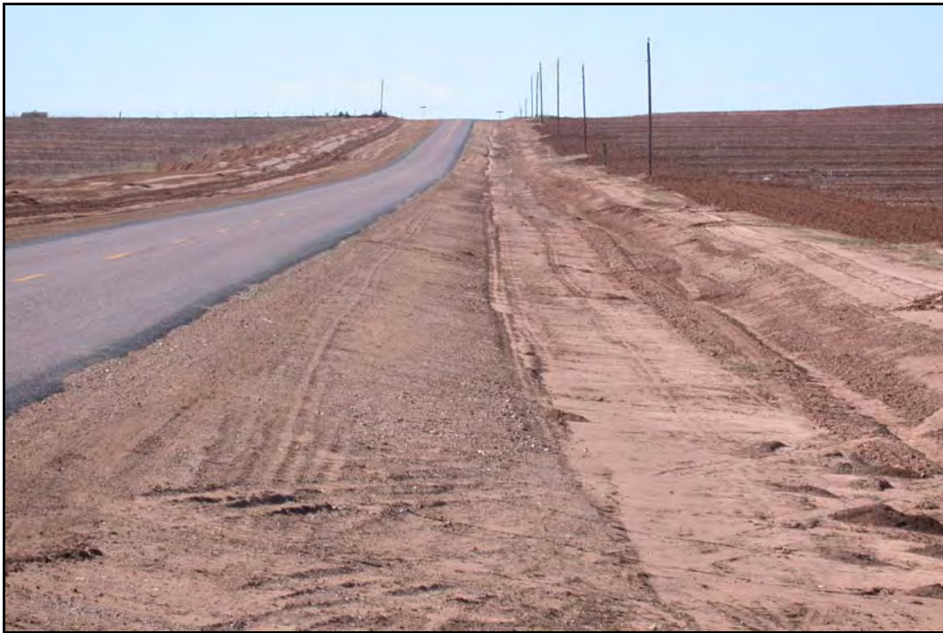
FIG 5.23 Reshaping (Pulling) Shoulders, Childress District (see Childress District Profile, Photo 15)
