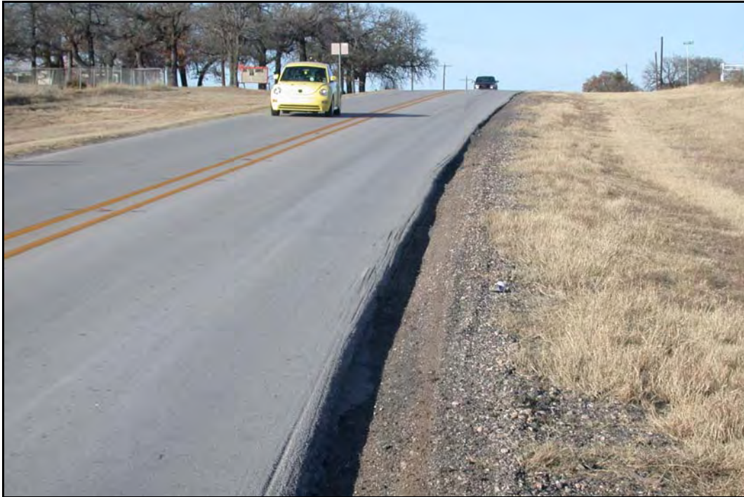
FIG. 4.8. Edge Drop-off at Relatively High-Volume, Narrow FM Road (21-foot width, ADT 4,400 vehicles/day).
