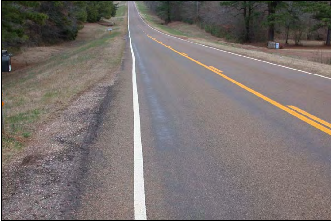
FIG 5.20 Inverted Profile Pavement Marking, Atlanta District (see Atlanta District Profile, Photo 27)
