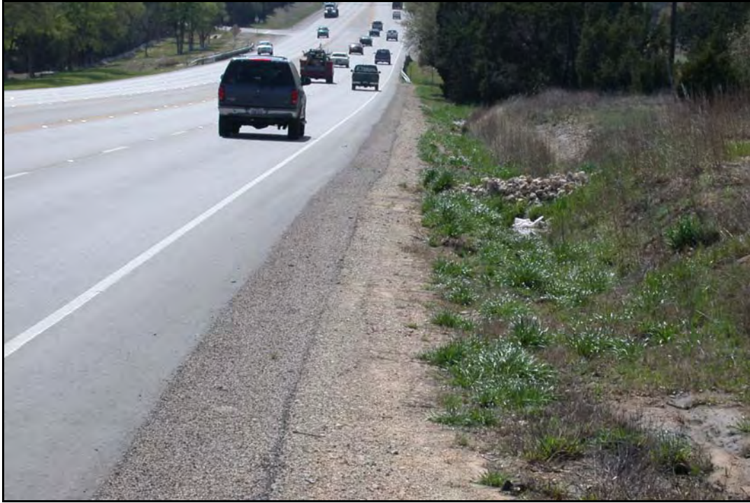
FIG. 5.29 Strip Seal Coat on a Contract Replenishing Project Using Flex Base, Austin District (see Austin District Profile, Photograph 4)
