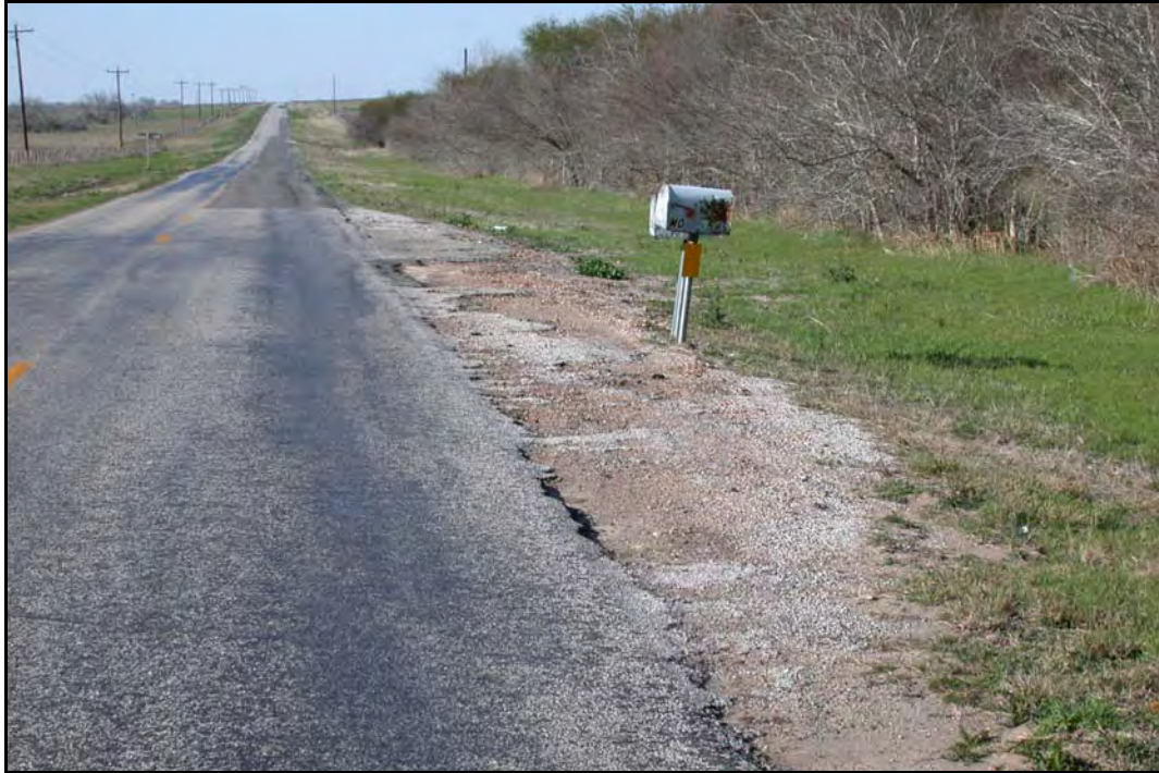
FIG. 4.14. Typical Edge Drop-off at Mail-box Turnout.
