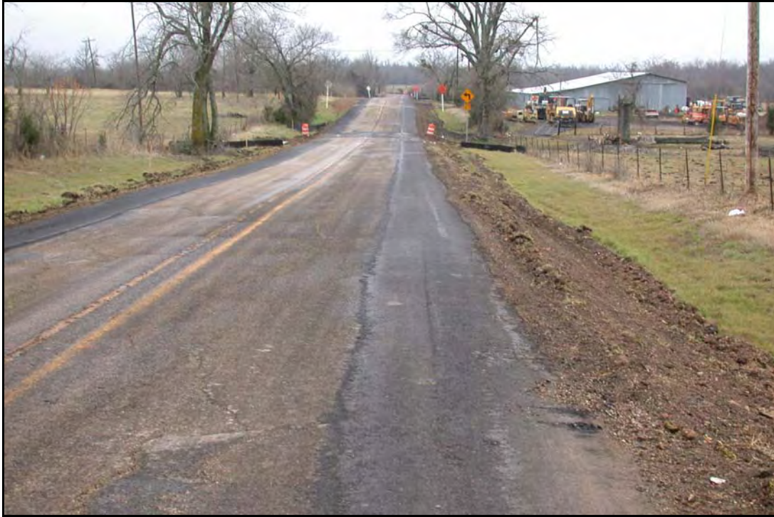
FIG. 6.9 FM 194 Contract Road Widening, Paris District (see Paris District Profile, Photo 30)
