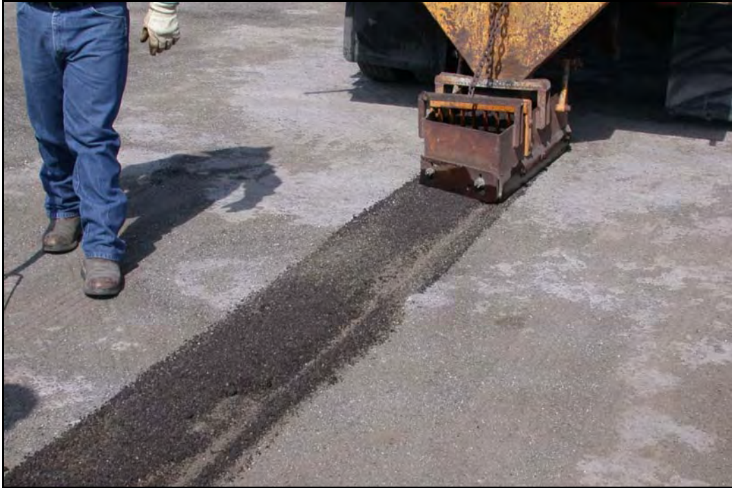
FIG. 5.33 Limestone Rock Asphalt (LRA) for Pavement Edge Repair, Pharr District, (see Pharr District Profile, Photograph 7)
