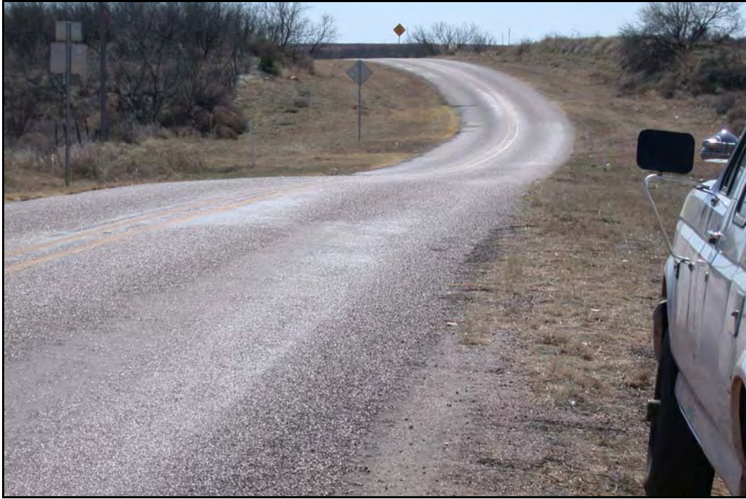
FIG. 4.4. Typical Narrow FM Road in West Texas
