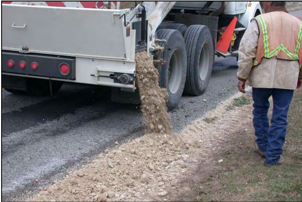
FIG. 5.27 Delivering Flex Base to the Pavement Edge Using a Swenson Tailgate Cross Conveyor (a.k.a. “Swenson Spreader”), Brownwood District (see Brownwood District Profile, Photo 13)
