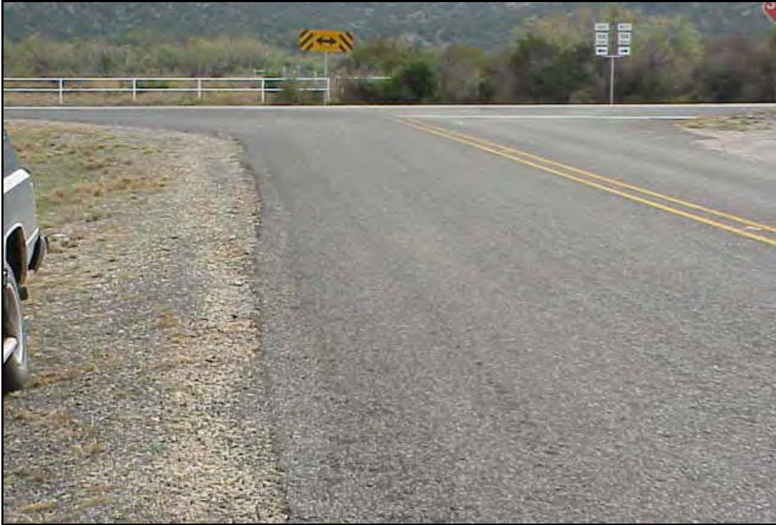
FIG. 6.13. RM 2059 Road Widening, Coke County Texas, San Angelo District (see San Angelo District Profile, Photo 14)
