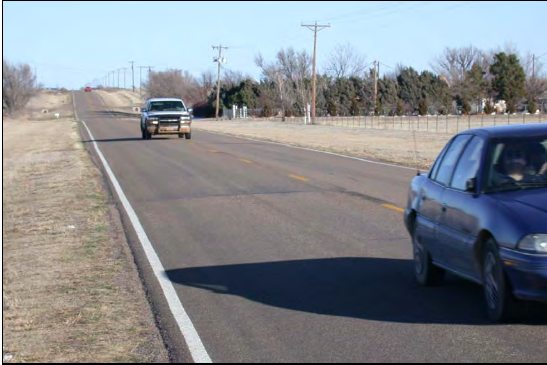
FIG. 6.15. FM 1151 Road Widening, Armstrong County Texas, Amarillo District (see Amarillo District Profile, Photo 29)
