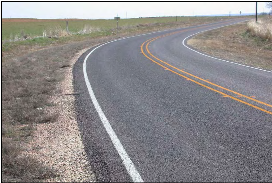
FIG. 6.8 FM 670 Contract Road Widening, Abilene District (see Abilene District Profile, Photo 7)
