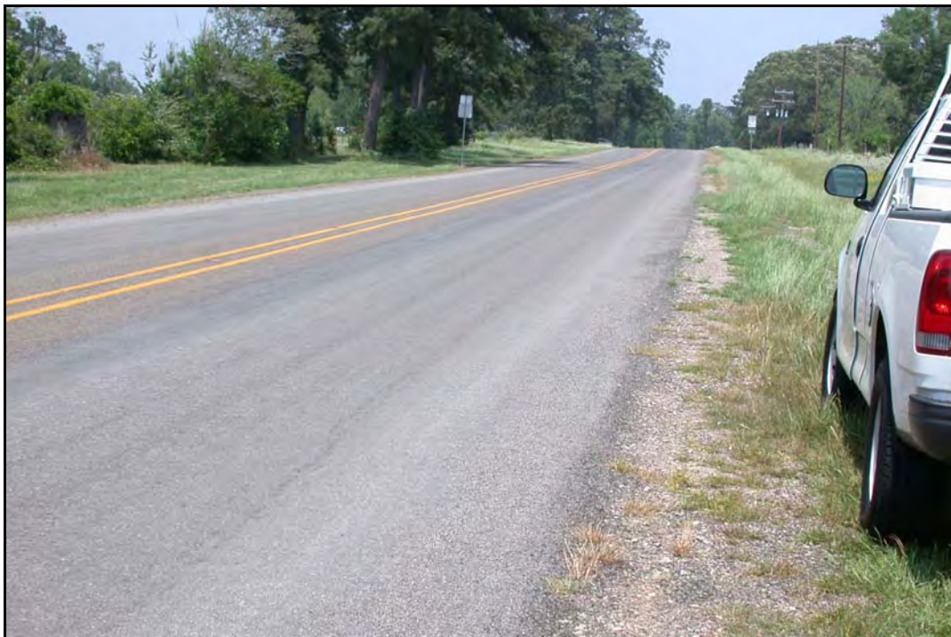
FIG. 6.16. FM 1005 Road Widening, Jasper County Texas, Beaumont District (see Beaumont District Profile, Photo 3)
