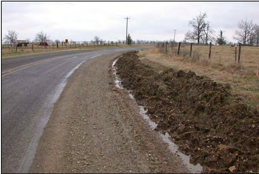
FIG. 5.26 Replenishing Repair at the Inside Horizontal Curve of an FM Road, Paris District (see Paris District Profile, Photo 23)
