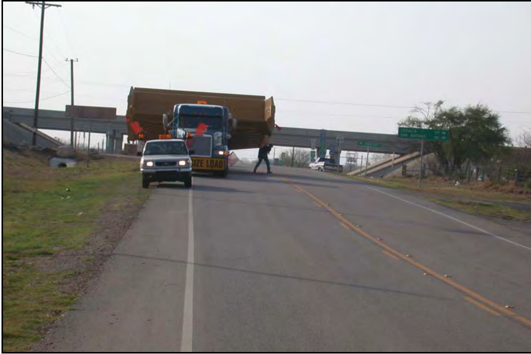
FIG. 4.9. Edge Damage due to Unconventional Traffic.
