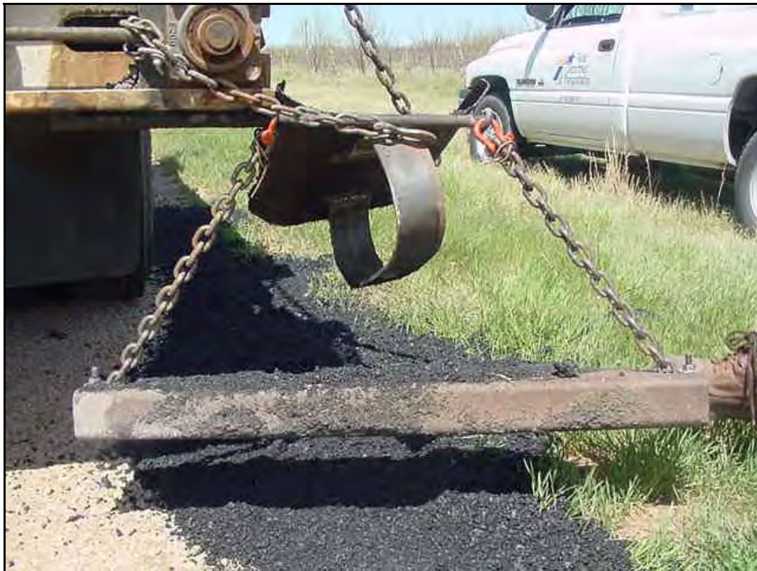
FIG. 7.16 Close-up View, Side Discharge Chute and Tow-Behind Drag Bar for Edge Repair, Wichita Falls District
