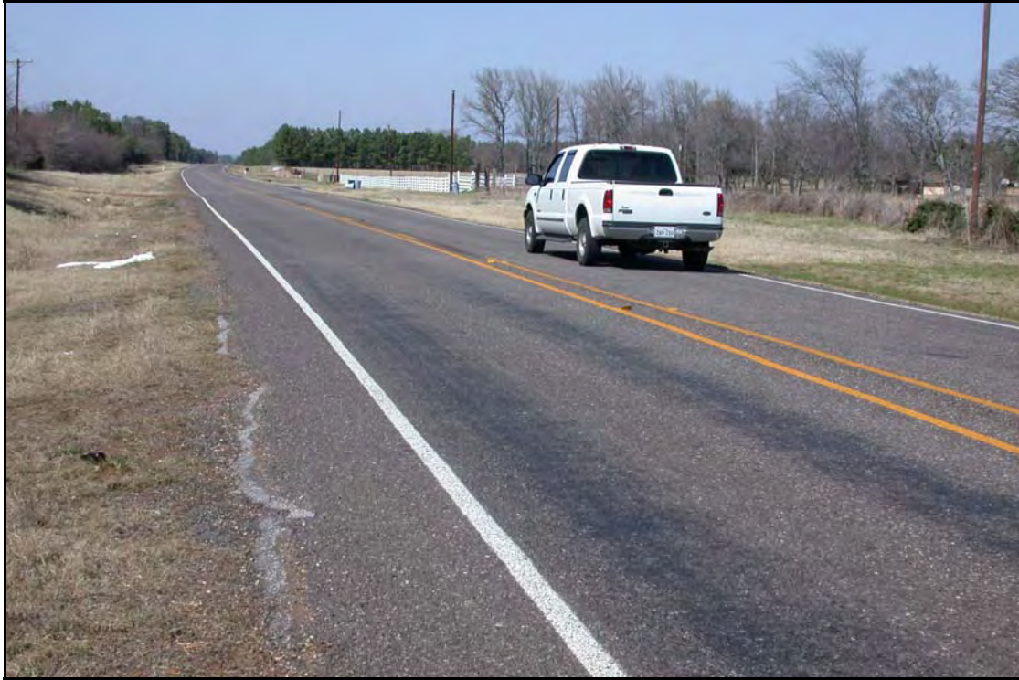
FIG. 6.19. FM 2661 Road Widening, Smith County Texas, Tyler District (see Tyler District Profile, Photo 8)
