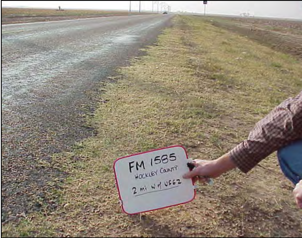
FIG 5.15 Encroachment of Vegetation onto the Pavement Edge, Lubbock District (see Lubbock District Profile, Photo 16)
