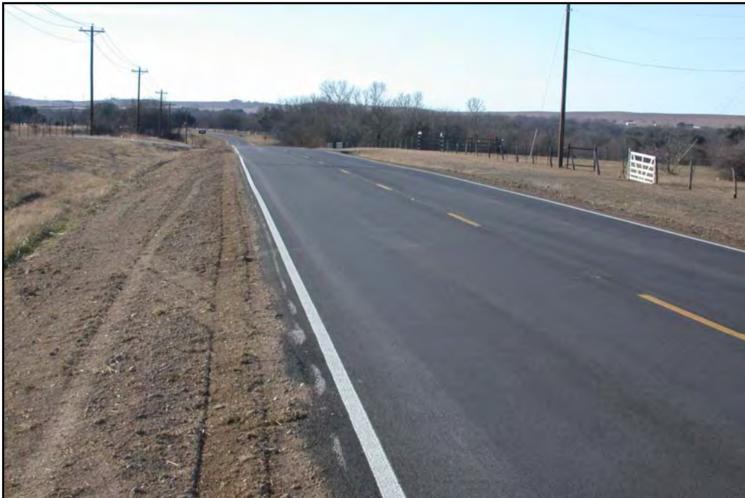
FIG 5.18 Typical Striping, Low-Volume FM Road, Fort Worth District (see Fort Worth District Profile, Photo 6)
