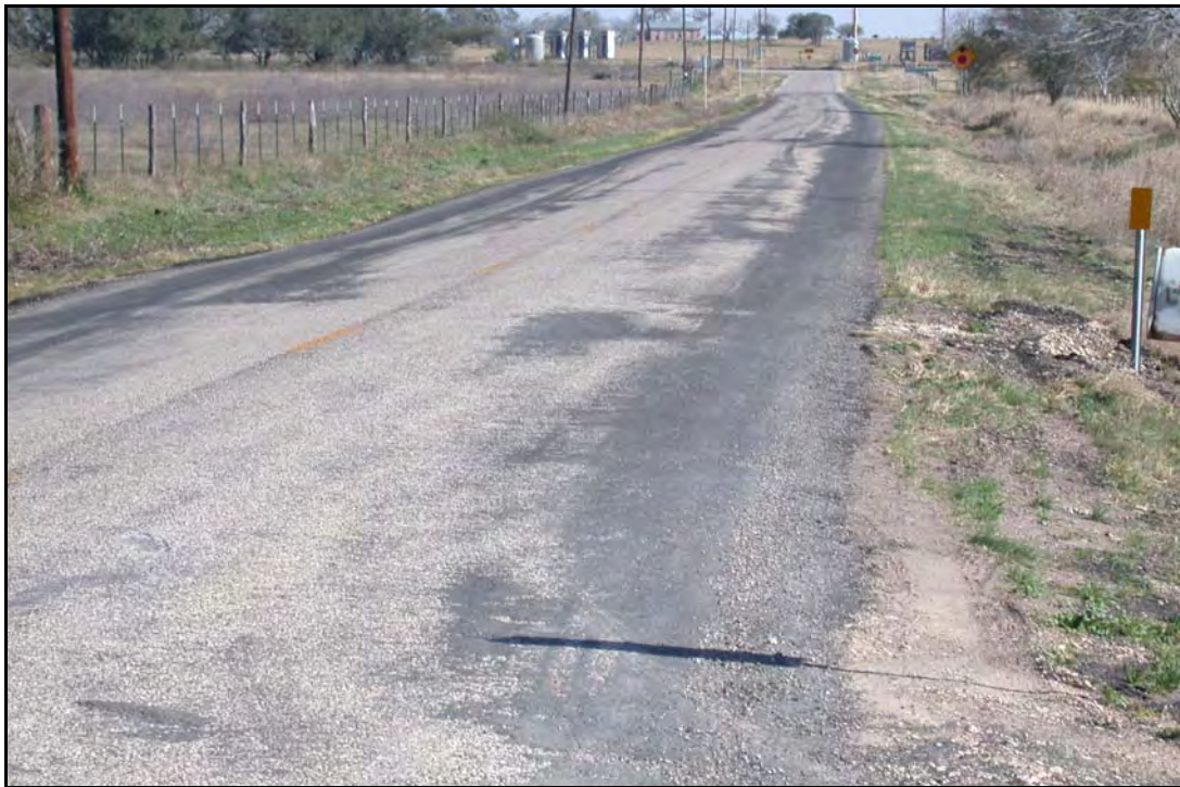
FIG. 6.14. FM 239 Road Widening, DeWitt County Texas, Yoakum District (see Yoakum District Profile, Photo14).
