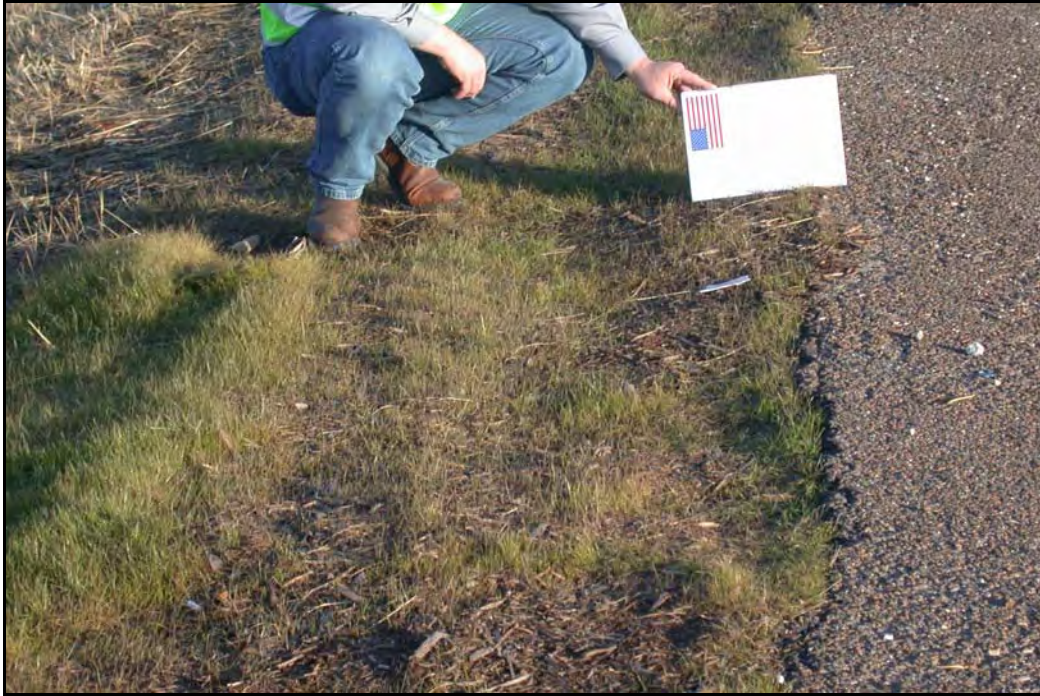
FIG 5.12 Composting to Promote Vegetation Growth, Fort Worth District (see Fort Worth District Profile, Photo 48)
