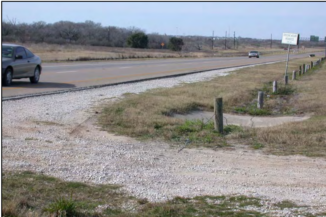
FIG 5.16 Post and Cable Median Barrier, San Antonio District (see San Antonio District Profile, Photo 15)
