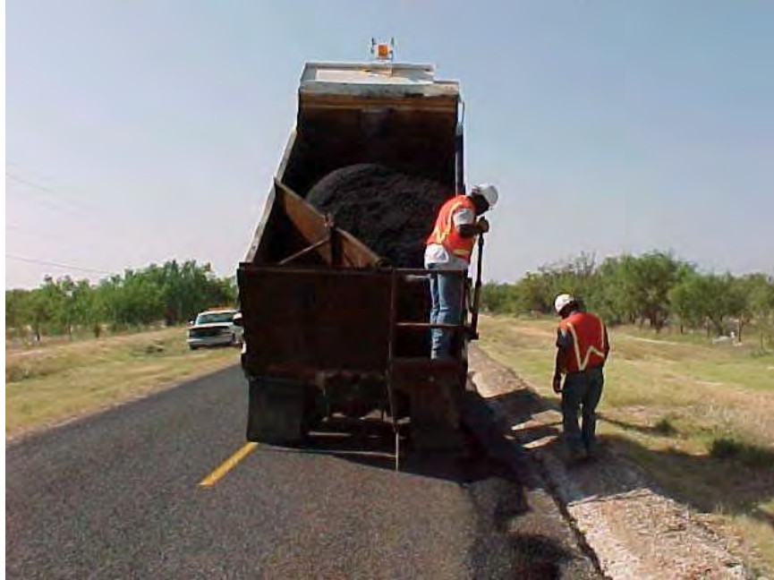
FIG. 7.13 Plywood Insert in Dump Truck Bed to Direct Flow of Material to Side-Discharge Chute, Abilene District ( Photo courtesy of Jones County Maintenance )
