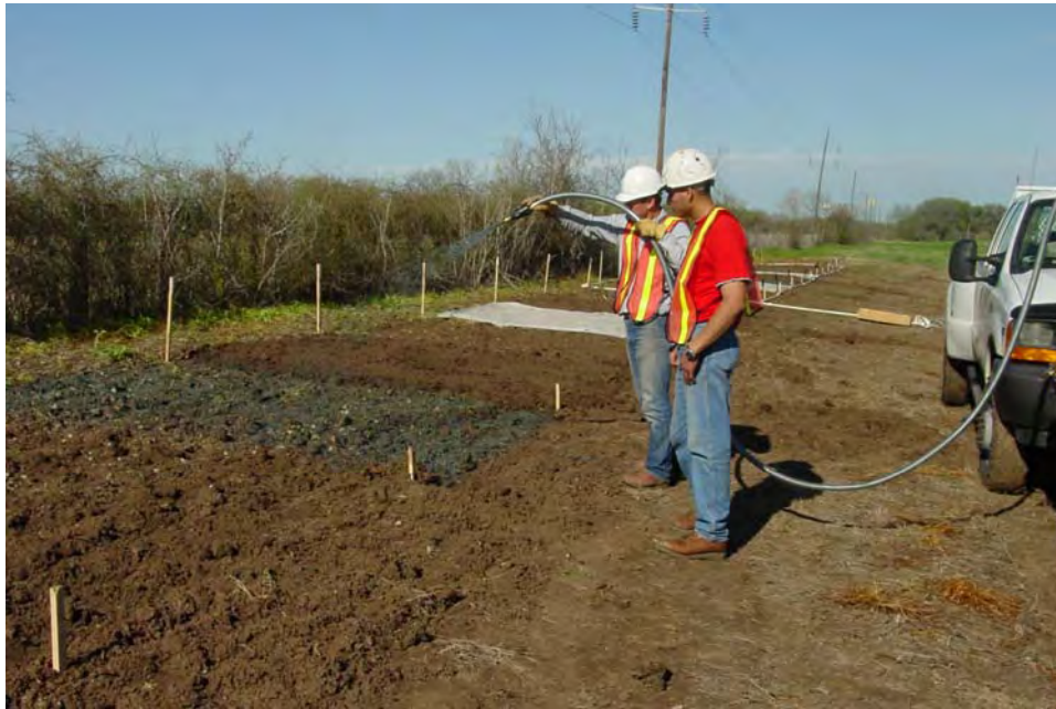
Figure 4.3 Application of Cellulose Fiber Mulch at the Falls County Field Site
