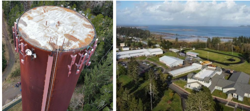
Figure 4-8 Critical infrastructure inspection drone aerial image: water tower (left) and School campus with tsunami VES (right; VES is building with flat roof and covered stairwells in each corner).
