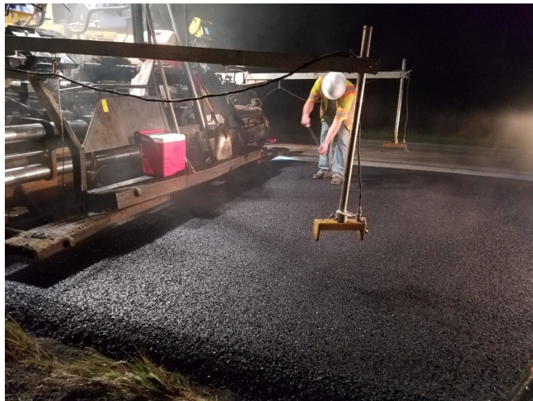
Figure 6-4. ECR SMA night paving on I-35 mainline in Spring of 2018
