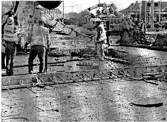
Figure 58 – Encasing existing utility
