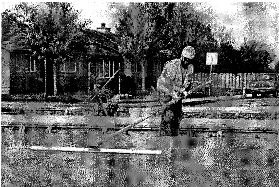
Figure 46 – Manual texturing of the pavement
