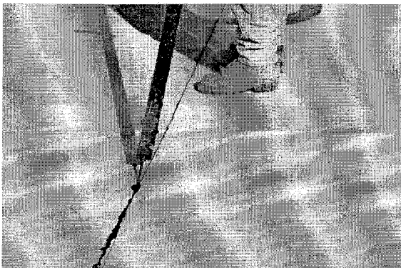
Figure 52 – Cleaning the joint reservoir
