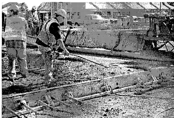
Figure 36 – Vibrating concrete
