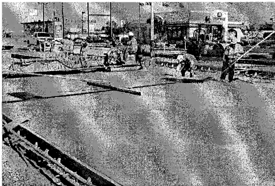
Figure 44 – Floating behind Whiteman screed
