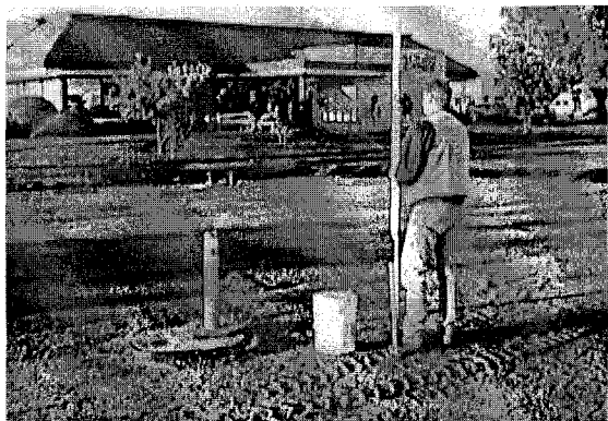
Figure 22 – Surveying the grade
