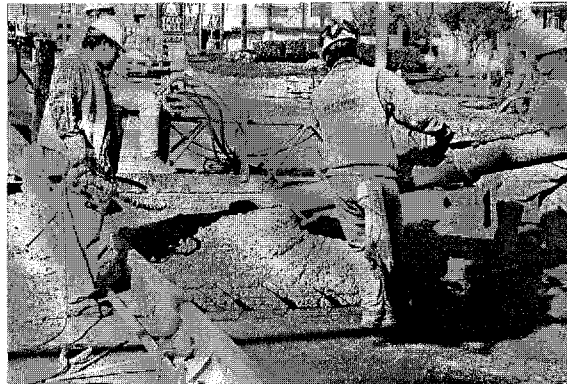
Figure 32 – Concrete discharge and paving operation
