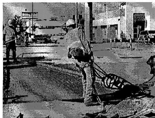
Figure 34 – Placement with roller screed
