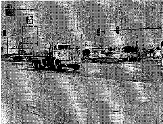
Figure 66 – Cleaning the roadway with water truck
