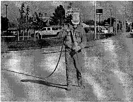
Figure 52 – Cleaning the joint reservoir
