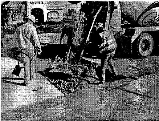
Figure 62 – Placing concrete for backfill
