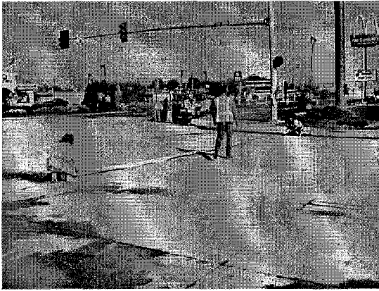
Figure 70 – Placing stopbar and lane striping
