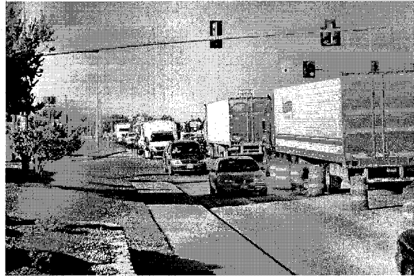
Figure 7 – Traffic flow pushed to the west during construction of approach legs
