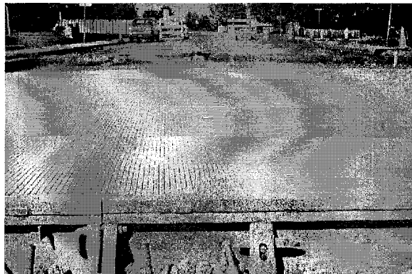
Figure 47 – Tines of freshly placed concrete
