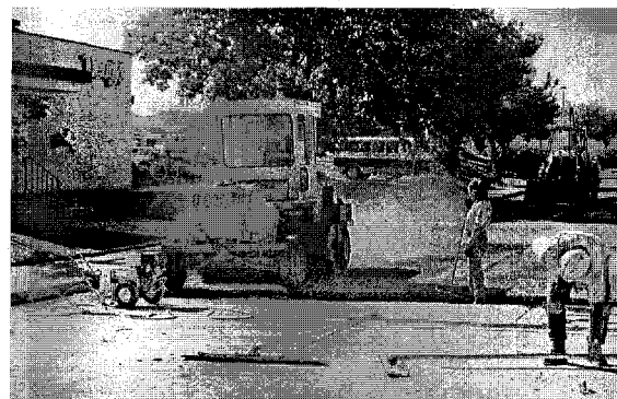
Figure 65 – Brooming preparation for ACP
