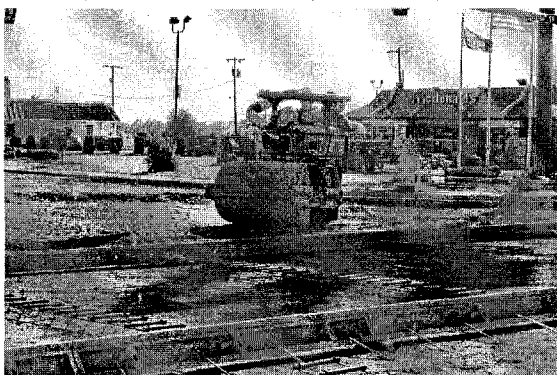
Figure 24 – Rolling grade
