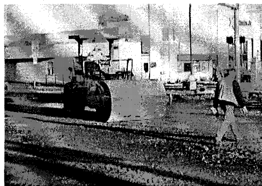
Figure 25 – Subgrade compaction
