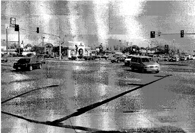
Figure 15: The Intersection of SR 395 and Kennewick Avenue prior to construction
