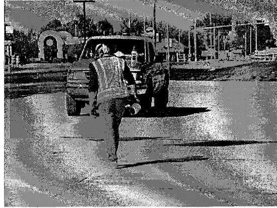
Figure 70 – Placing stopbar and lane striping
