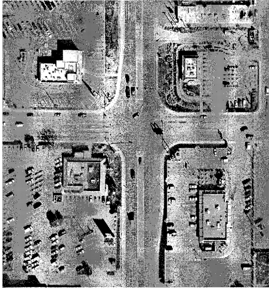
Stage 1: Construction of the left hand turn lane
