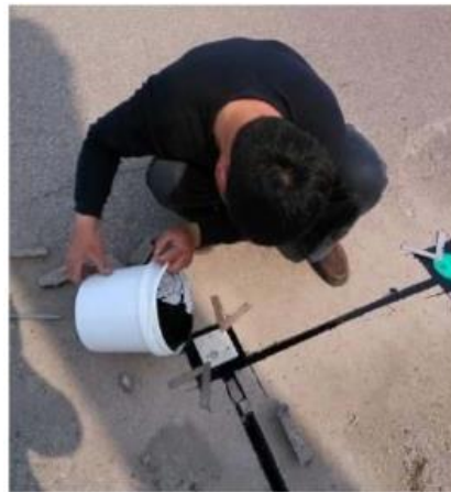
Figure 16. Embedded pavement sensor
