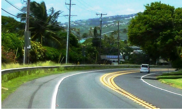
Figure 7. Roadway departure countermeasures applied at this curve include wider lane separation to prevent head-on collisions in the curve, raised pavement markers, widened shoulders, and a guardrail. Credit: FHWA.
