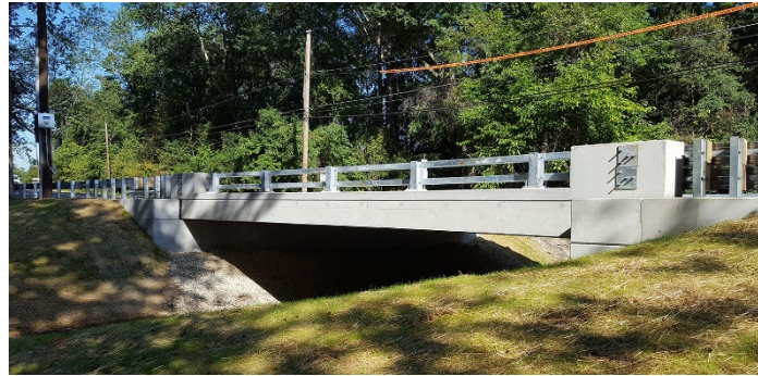
Figure 8. Delaware DOT combined precast elements with UHPC connections and a UHPC overlay on an Accelerated Innovation Deployment Demonstration project.
