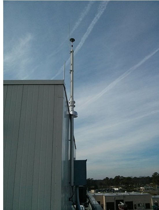
Figure 13 GPS and 1090MHz antennas on roof of William J Hughes Technical Center Federal Laboratory (WJHTC), Building #27
