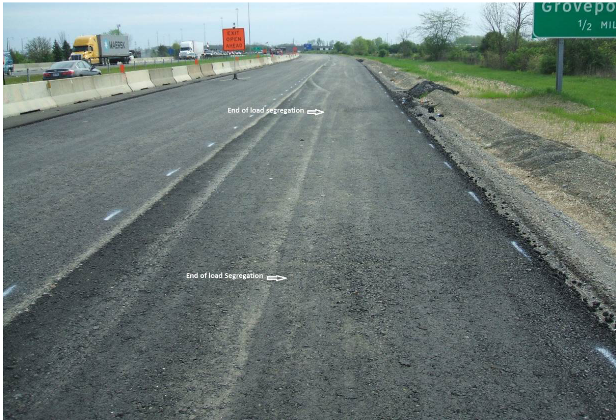
Figure 11-8. End of load segregation.
