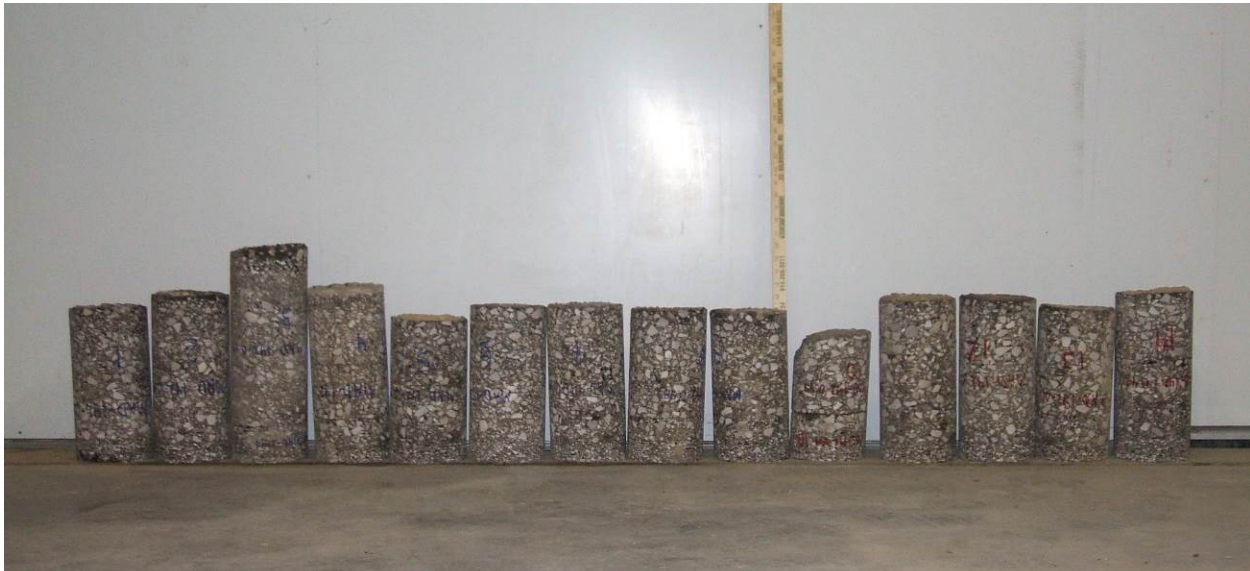
Figure 11-12. Pavement specimen cores from MAD-142.
