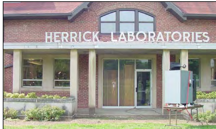
Figure 3.2: Experimental set-up at Herrick Labs, Loudspeakers directed at set of two large and two small windows.
