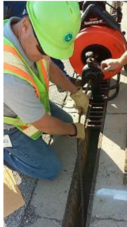
Figure 2.7. Use of mechanical drain in cleaning trench drains
