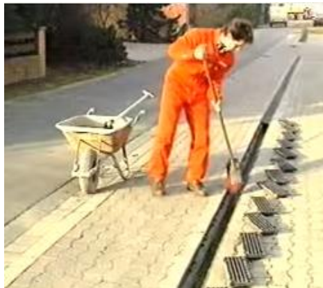
Figure 2.15. Manual Cleaning of Trench drains
