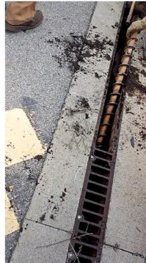
5- Disconnect auger section from drill
