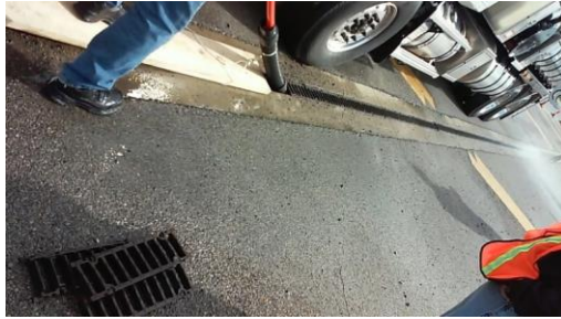
Figure 2.13. Reduced splashing when using Flounder nozzle
