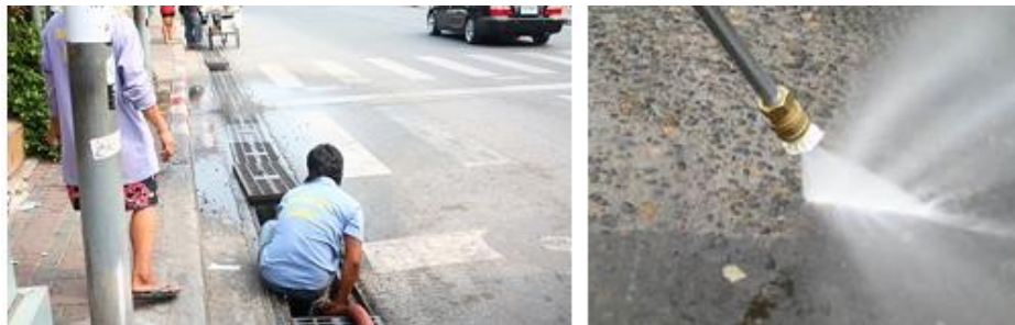
Figure 2.16. Cleaning Trench Drains by Flushing with Water
