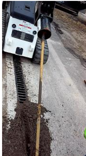
Figure 5.11. Debris collected near cleanout position
