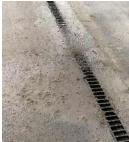
Figure 5.14. Water splash caused when a sewer truck is used for cleaning the drain
