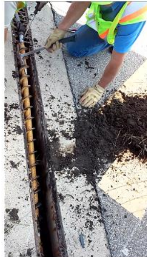
5- Disconnect auger section from drill
