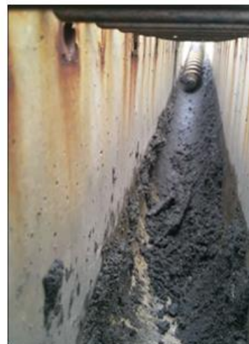
After Cleaning with HDD
