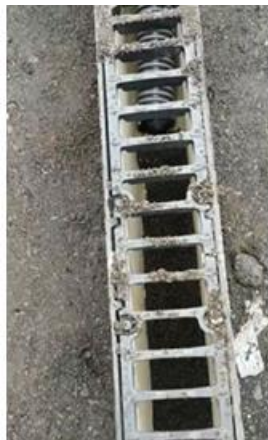
Before Cleaning with Hurricane 500
