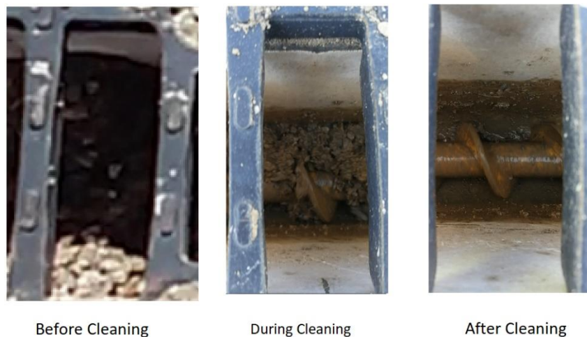
Figure 5.28. Results of cleaning trench drain with HB unit, augers and vacuum
