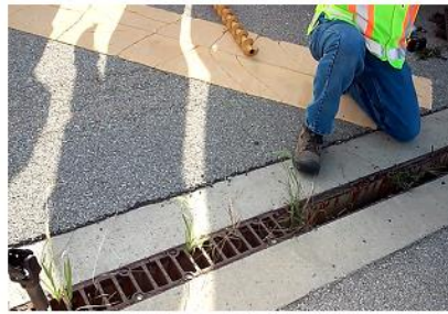
2-Remove grates from some drain's sections
