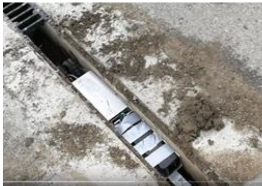
Figure 5.13. UC robot inside the trench drain
