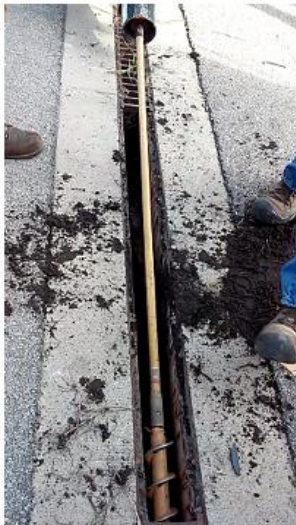
4-Push auger section forward with drill
