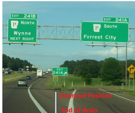
Figure 4.3. Use of trench drains in highway gore areas
