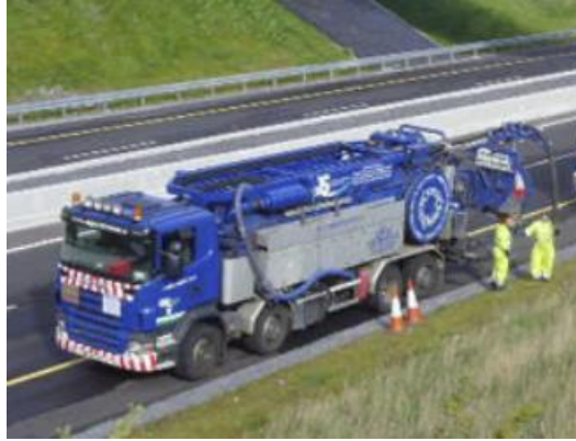
Figure 2.19. Cleaning a Trench Drain by a Vactor-jet
