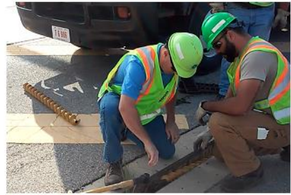
3-Insert first auger section into drain
