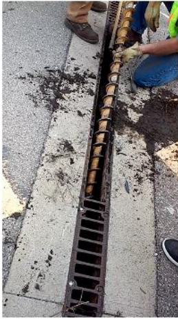
6-Connect another auger section to previous section and to drill
