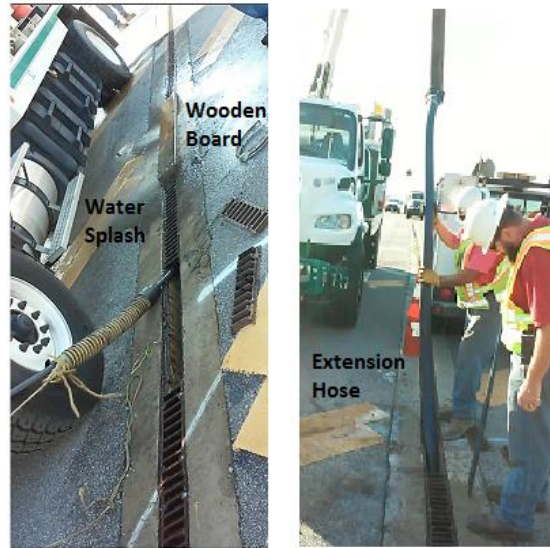
1-Placing Nozzle in Drain
