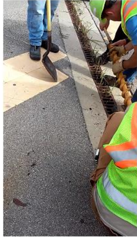
6-Connect another auger section to previous section and to drill
