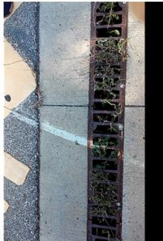
Before Cleaning with HDD
