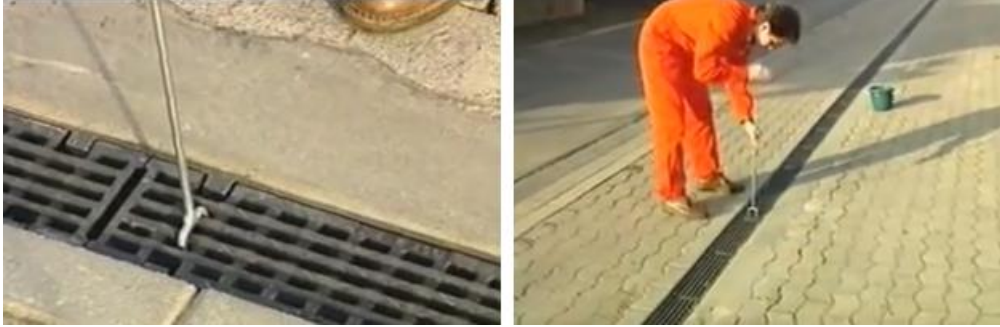
Figure 2.4. Tool to remove grates attached with locking rods
