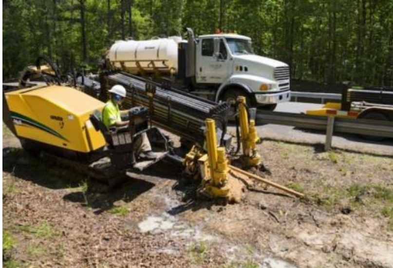
Figure 2.21. Installing pipes using a HDD rig
