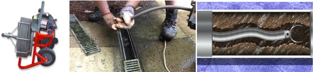
Figure 2.17. Cleaning a Trench Drain by a Mechanical Drain Cleaner
