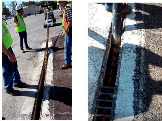
Figure 5.26. Use of HAB machine in conjunction with suction excavator
