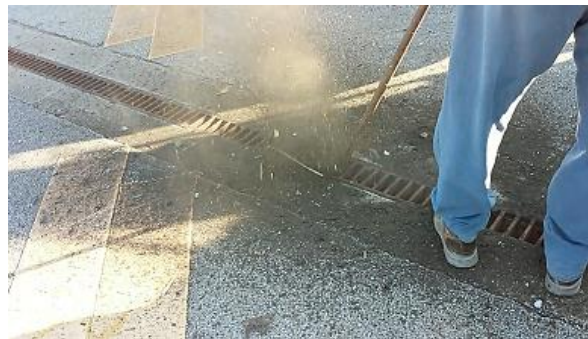
Figure 2.6. Use of compressed air in cleaning drains
