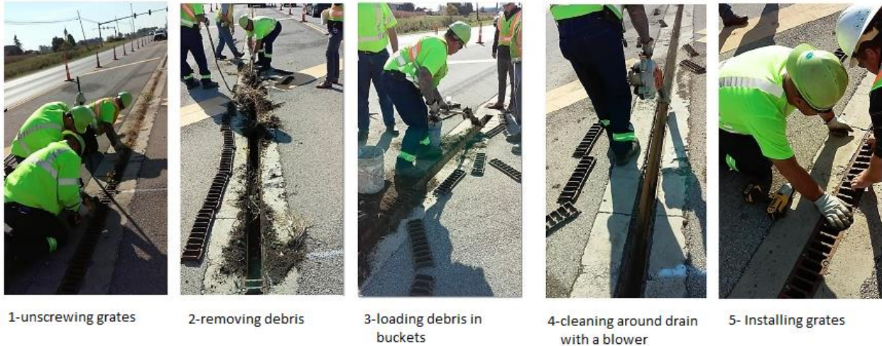
Figure 2.5. Manual cleaning of trench drains
