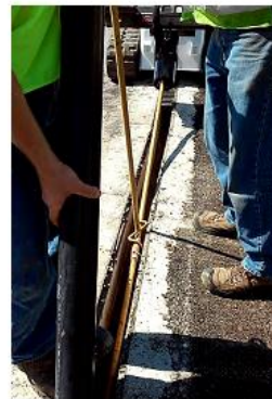
Figure 5.25. Use of drill rod guide
