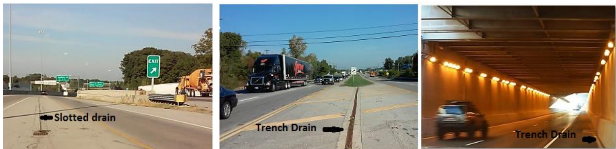
Figure 2.1. Various installations of trench and slotted drains in Franklin County, Ohio
