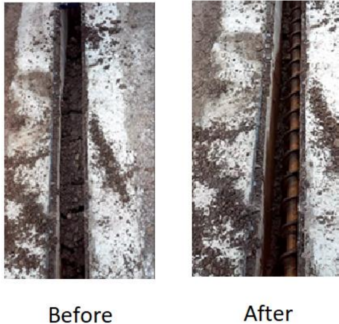
Figure 5.10. Results of cleaning trench drain with HAB and augers
