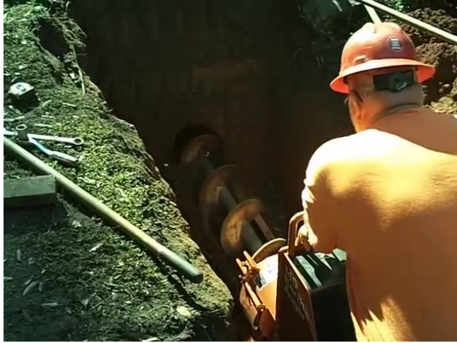
Figure 2.22. Horizontal Auger Boring
