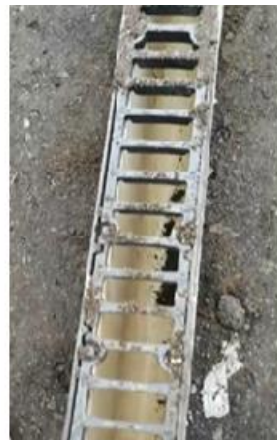
After Cleaning with Hurricane 500
