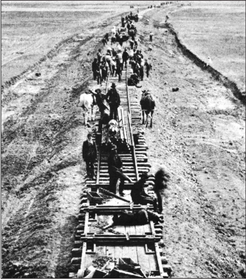
Construction forces pushing westward from Minot, 1867. A record of 8 ½ miles of track was laid on August 11, 1887.
