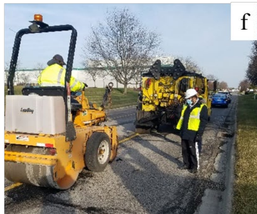
Figure C.8 Equipment used during the installation of patch: a) hot box used by the City of Columbus, b) hot box used by City of Cleveland, c) equipment used by City of Columbus for spray injection, d) equipment used by City of Cleveland for spray injection, e) tamper used for compaction, f) a five ton roller for compaction
