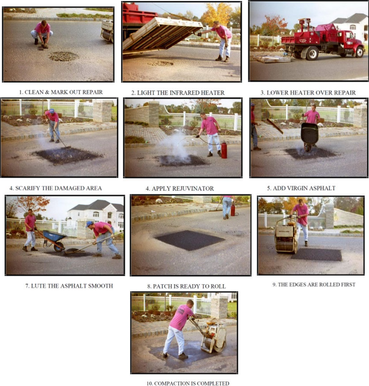
Figure B.7 Best practices corresponding to the method of tow-behind combination infrared asphalt heater/reclaimer
