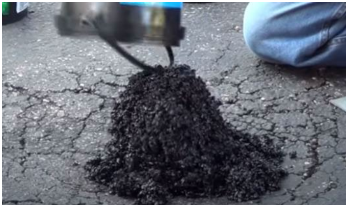
Figure B.3 Material placement recommended for throw-and-go method
