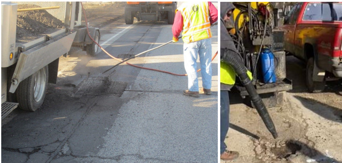
Figure B.2 Pothole preparation method of cleaning using compressed air
