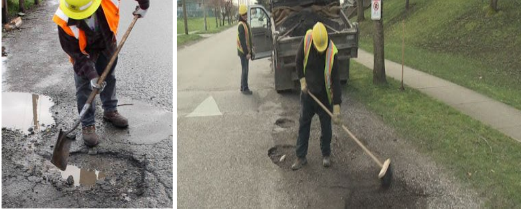
Figure B.1 Sweeping method for pothole preparation
