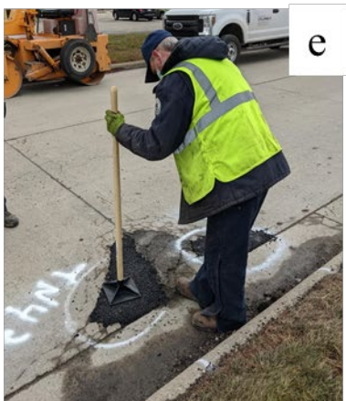
Figure C.8 Equipment used during the installation of patch: a) hot box used by the City of Columbus, b) hot box used by City of Cleveland, c) equipment used by City of Columbus for spray injection, d) equipment used by City of Cleveland for spray injection, e) tamper used for compaction, f) a five ton roller for compaction
