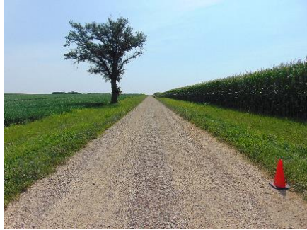
Figure 4. Typical gravel road.
