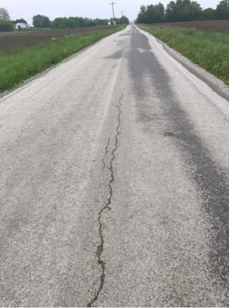
Figure C-8. Various distress with their severity levels recorded for seal coated Lester road in Williamsville Township.
