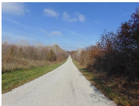
Figure 3. Typical seal-coated road.
