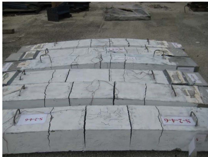
Figure 1-12 Cracking pattern in closure joints region.
