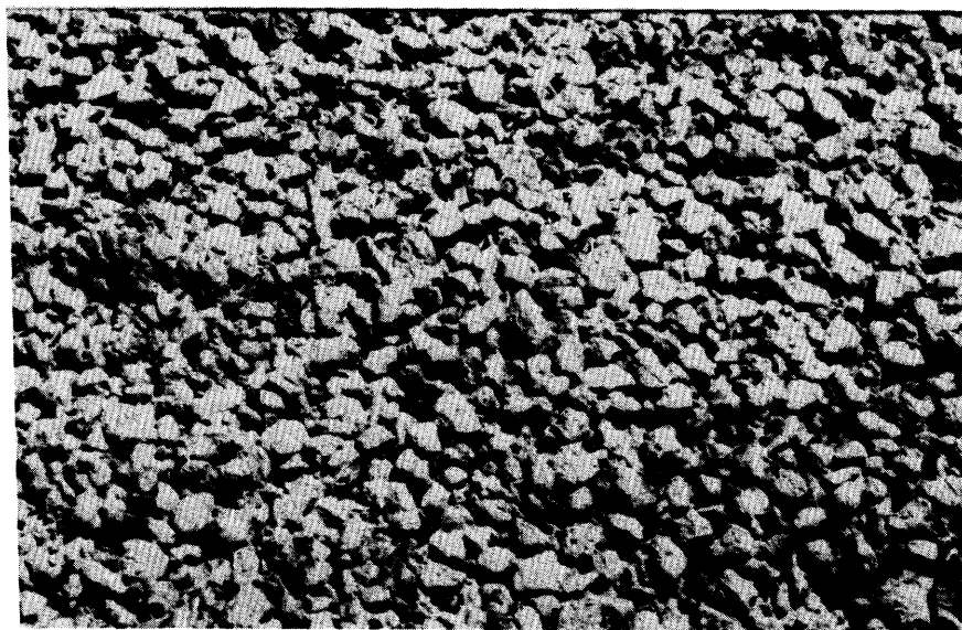
Photo No. 5. Cement-Treated Permeable Base
