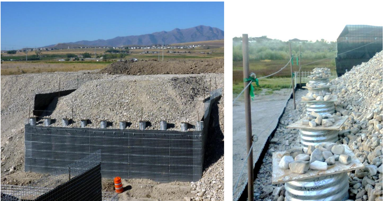
Figure 2-14: Piles in Corrugated Metal Sleeves near a Bridge Abutment
