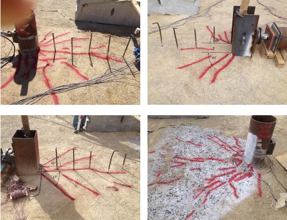
Figure 5-1: Failure Plane around the Piles: Round (top left), H (top right), Square (bottom left), Round in CMS (bottom right)
