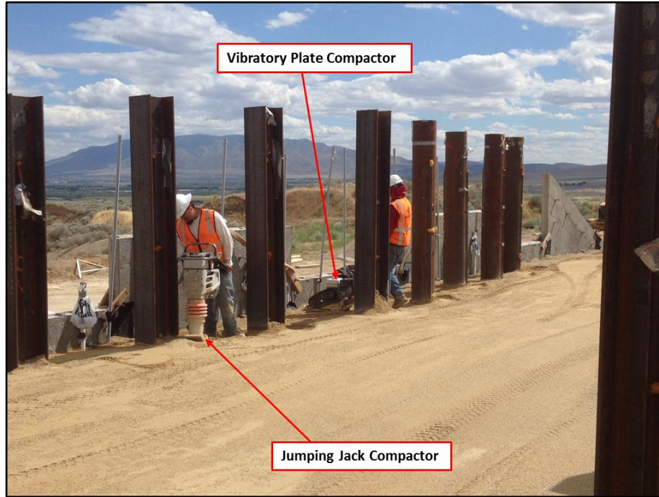
Figure 3-13: Compaction of backfill between the test piles and the back of wall using jumping jack and vibratory plate compactors.
