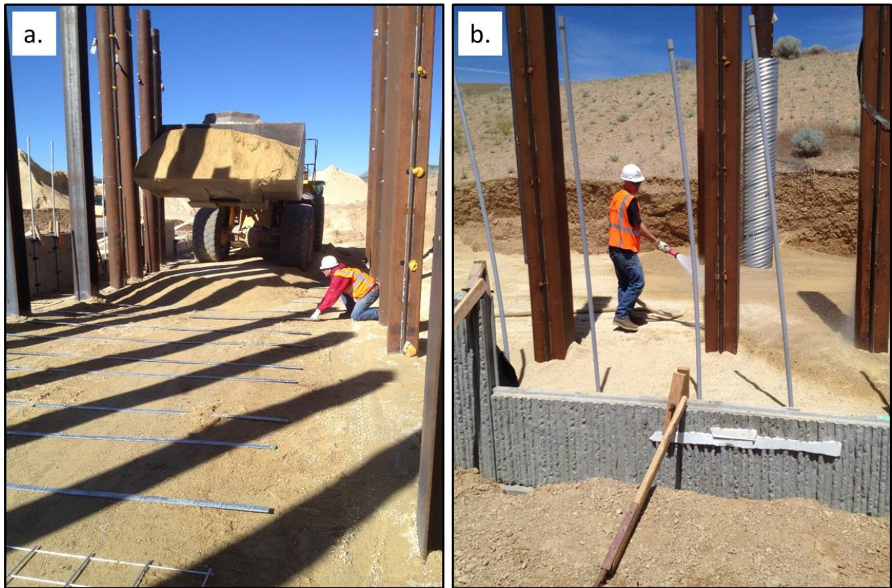
Figure 3-11: (a) Backfill lifts behind test piles; (b) moisture conditioning of backfill.
