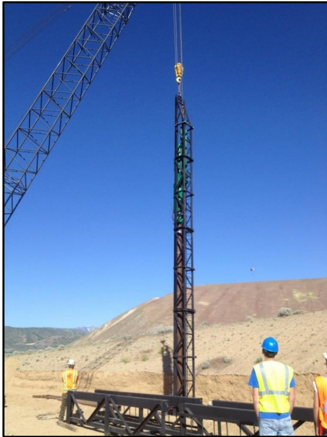
Figure 3-3: Installation of piles using a diesel hammer.
