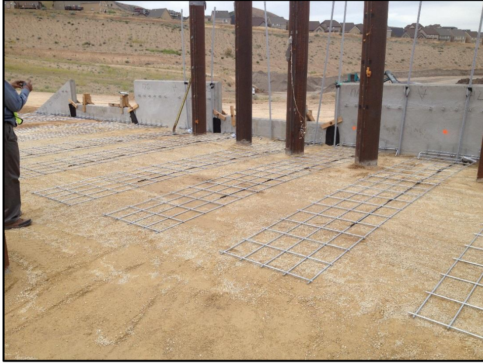
Figure 3-8: SSL galvanized steel welded-wire grid soil reinforcing layout with test piles.
