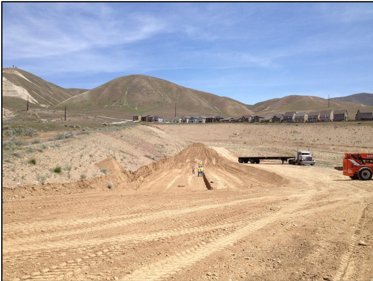
Figure 3-2: Project site after completion of site grading.
