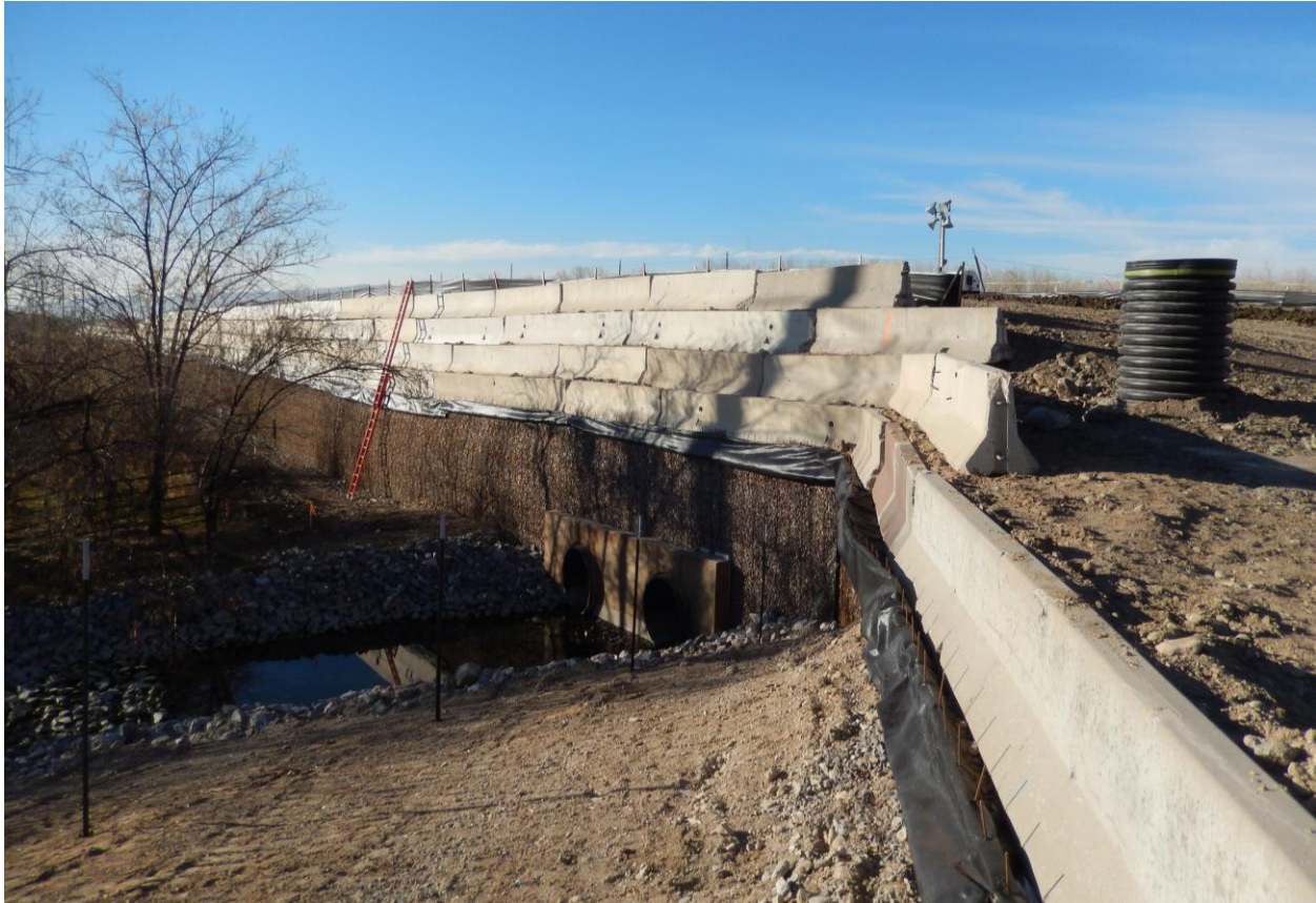
Figure 2-4 Full-height MSE wall and surcharge along the south side of the new roadway.
