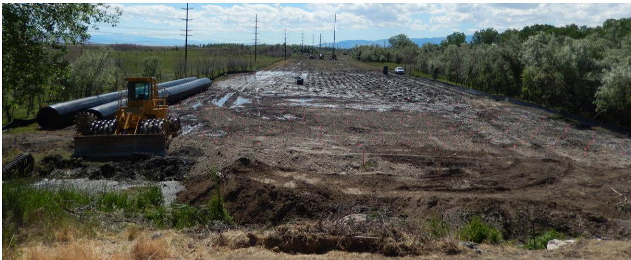
Figure 2-1 Provo Westside Connector site during PV drain installation.
