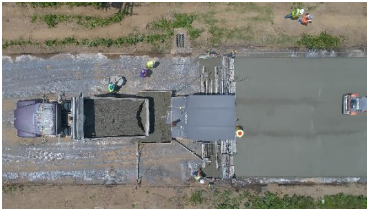
(e) Paving Operation
