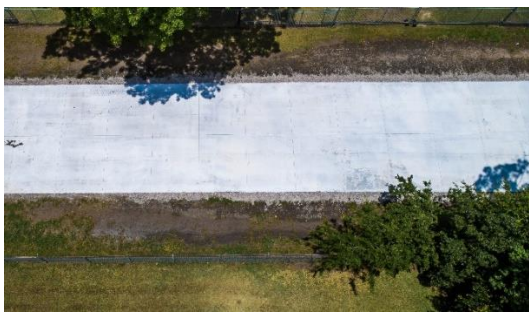
(h) Final surface after curing and saw-cut
