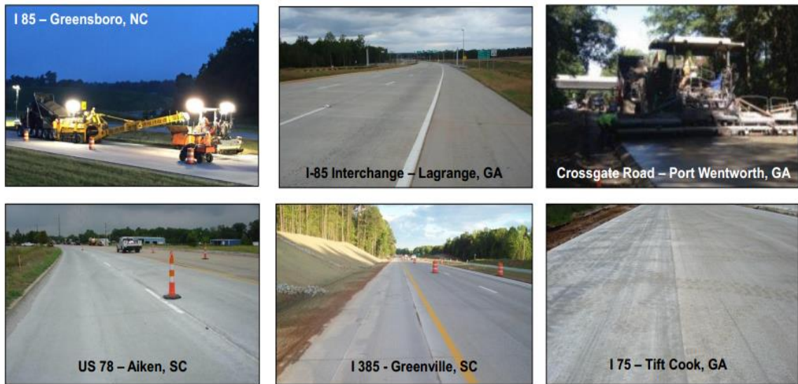
Figure 3. RCC application as shoulder and surface roads [31]
