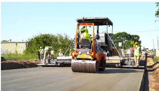
(f) Roller Compaction
