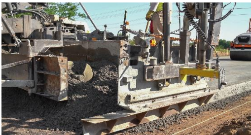
(c) Placement of RCC
