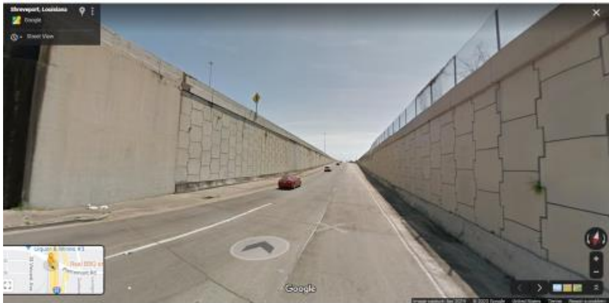
Figure 7. Mechanically Stabilized Earth (MSE) walls, Shreveport, LA
