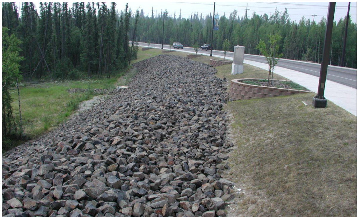
Figure 3-4 Photo Showing Test Section #1 and Ventilated Shoulder on Thompson Drive
