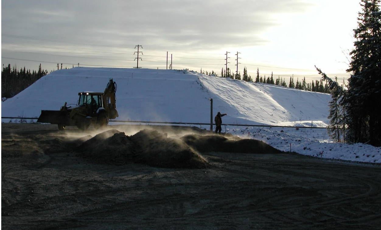
Figure 3-10 Winter Construction of Test Section #2
