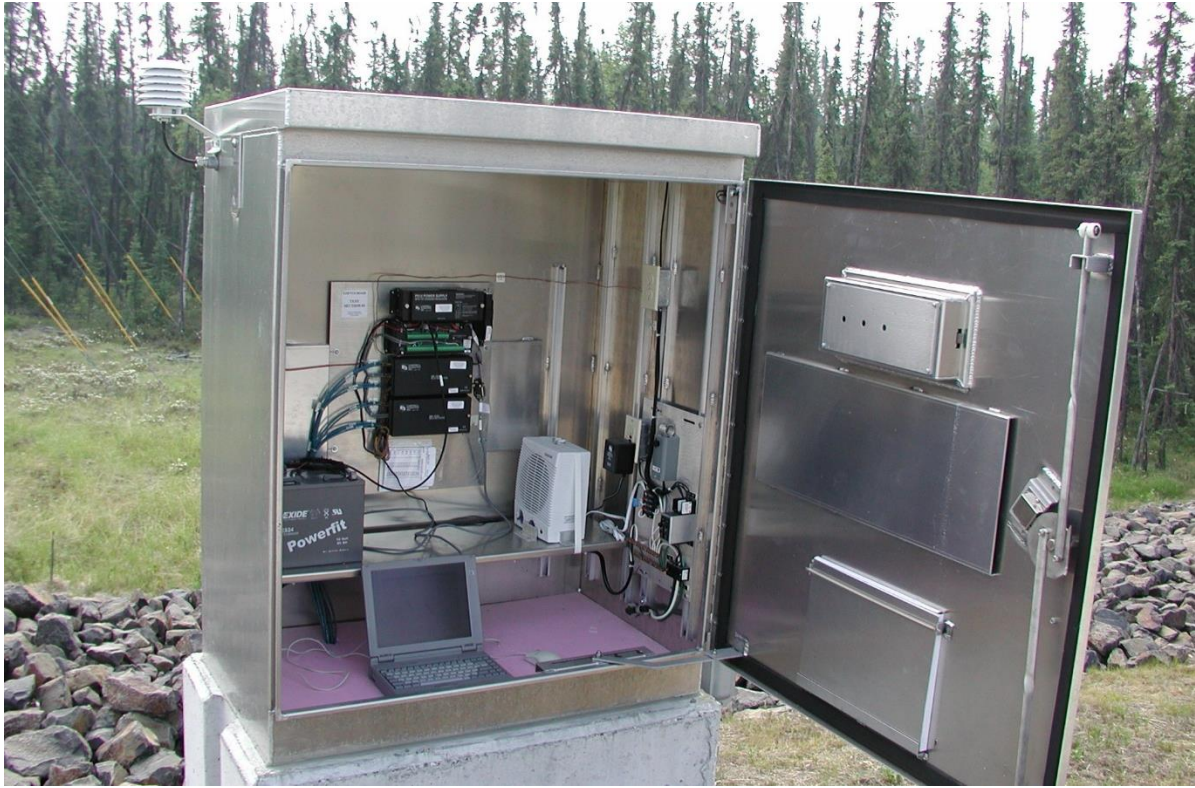
Figure 3-3 Data logging station for test section #1
