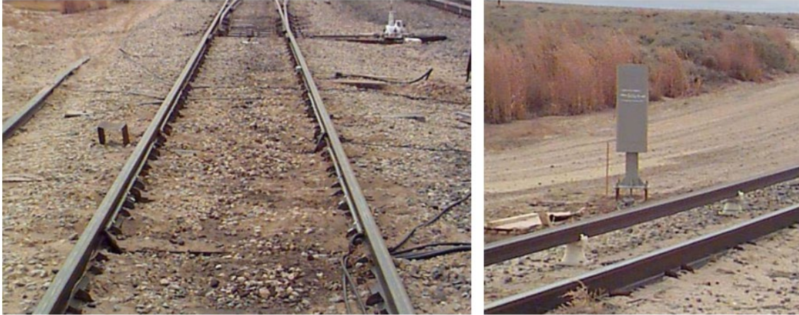
Figure 2.6 System 4 Inductive loop sensors (left) and radar detector for vehicle (right) (Reiff et al. 2003)
