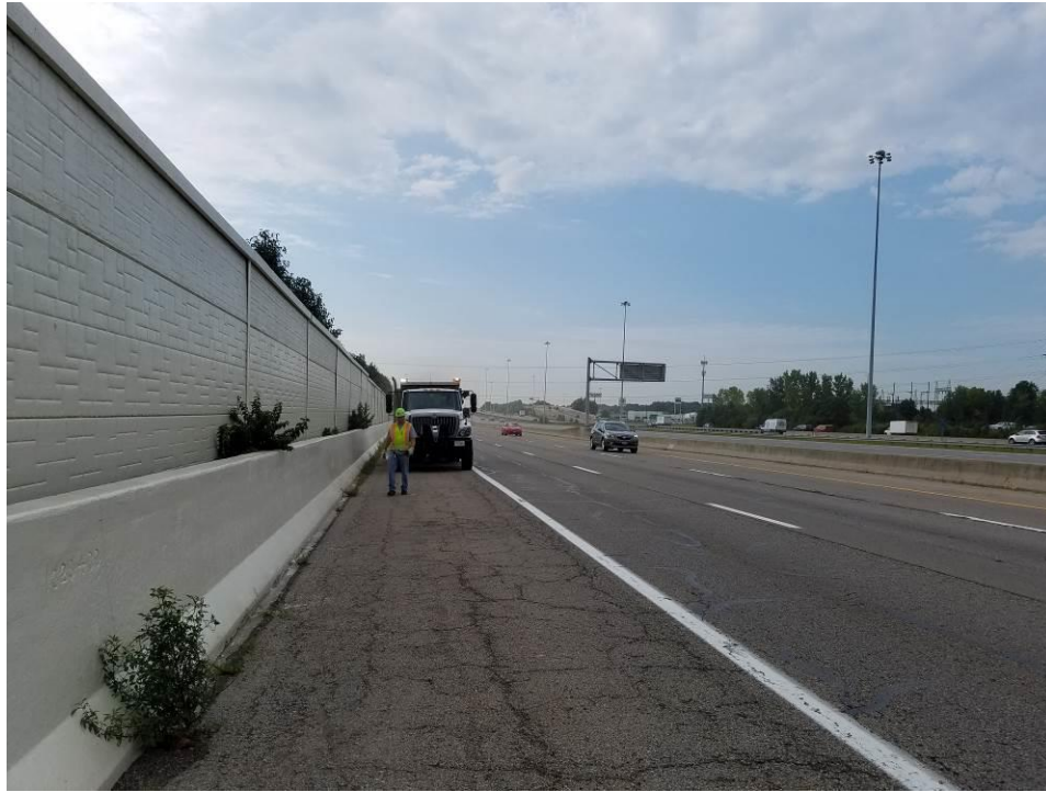
Figure 8.1 Clearing shoulder of large debris prior to sweeping
