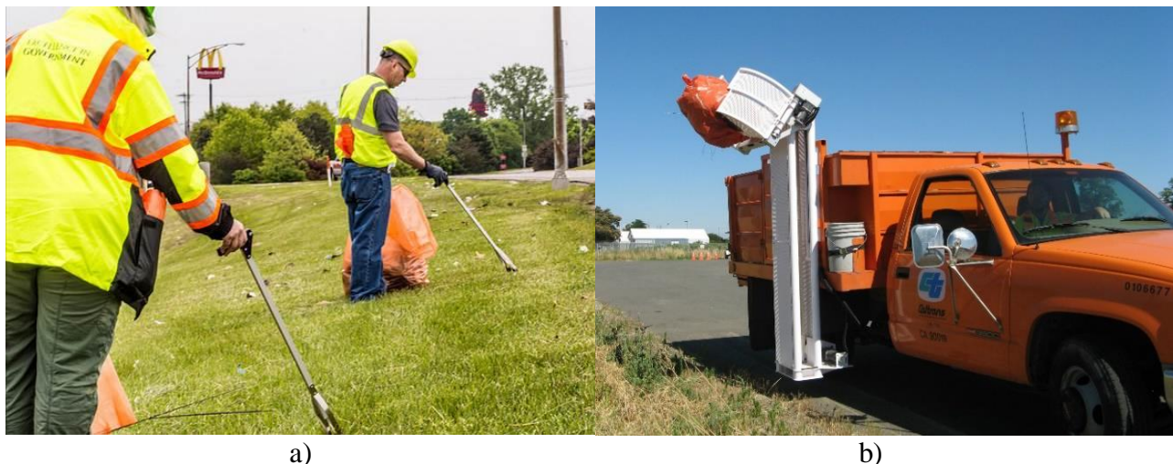
Figure 9.2 a) Manual Litter Pick-up [https://www.flickr.com/photos/ohiodot/albums] b) Debris Removal Attachment [AHMCT, 2011].
