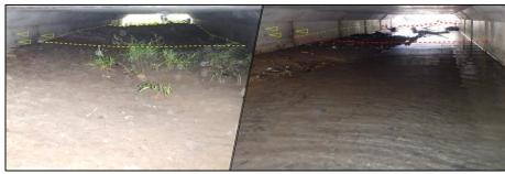
Top left) Aggraded sediment reduces capacity. Top middle) Installation of a culvert weir. Top left) Modeling results for culvert weir showing concentration of flow and shear stress in the right culvert after installing the culvert weir on the left culvert. Bottom left) Aggraded sediment prior to the installation of the culvert weir. Bottom right) Sediment following installation of culvert weir. Dashed line indicates sediment level prior to the maintenance activity.
