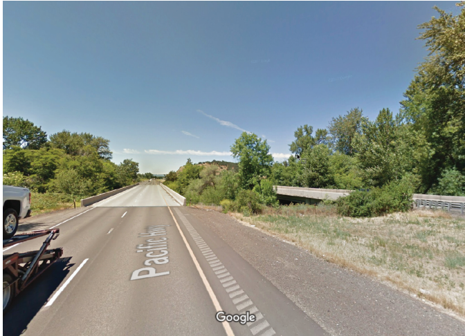
Figure 3. Photograph of Interstate-5 crossing of Bear Creek, Phoenix, Oregon. (Image capture June 2017, Google Maps, Street View. ©2018 Google, used with permission)
