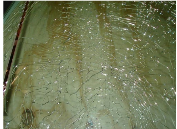
Fig. 4.16 Shattered exterior ply of cockpit windscreen [4.2].
