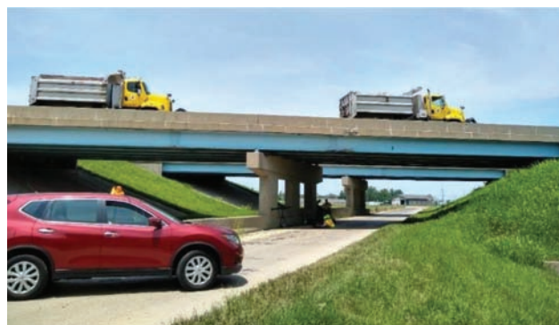
Figure 4.17 Load testing for Asset 037-55-05265.
