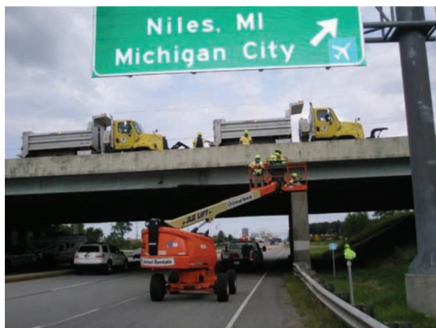
Figure 4.5 Load testing for Location 2. (Photograph courtesy of Prince Baah.)
