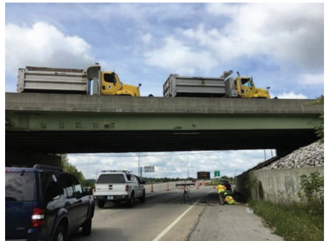
Figure 4.22 Load testing for Asset (45)46-53-05993.
