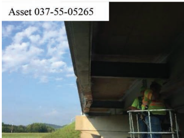
Figure 1.2 Damage to steel girders in the four bridges tested in this project.
