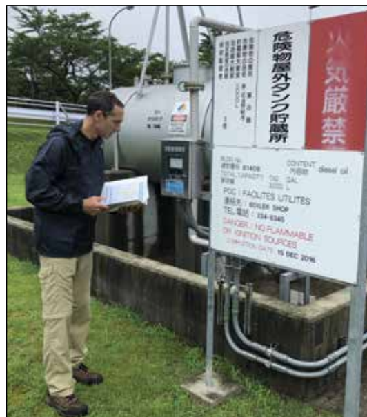
U.S. DOT Volpe Center Engineer, Richard Reiss, P.E., inspecting an aboveground fuel storage tank overfill prevention system component at Combined Arms Training Center Camp Fuji in Gotemba, Japan. (Image: U.S. DOT Volpe Center/ Richard Reiss)
