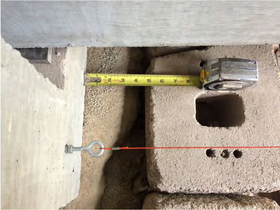
Figure A2.34 Corner of the abutment after all shaking motions for Test 1.
