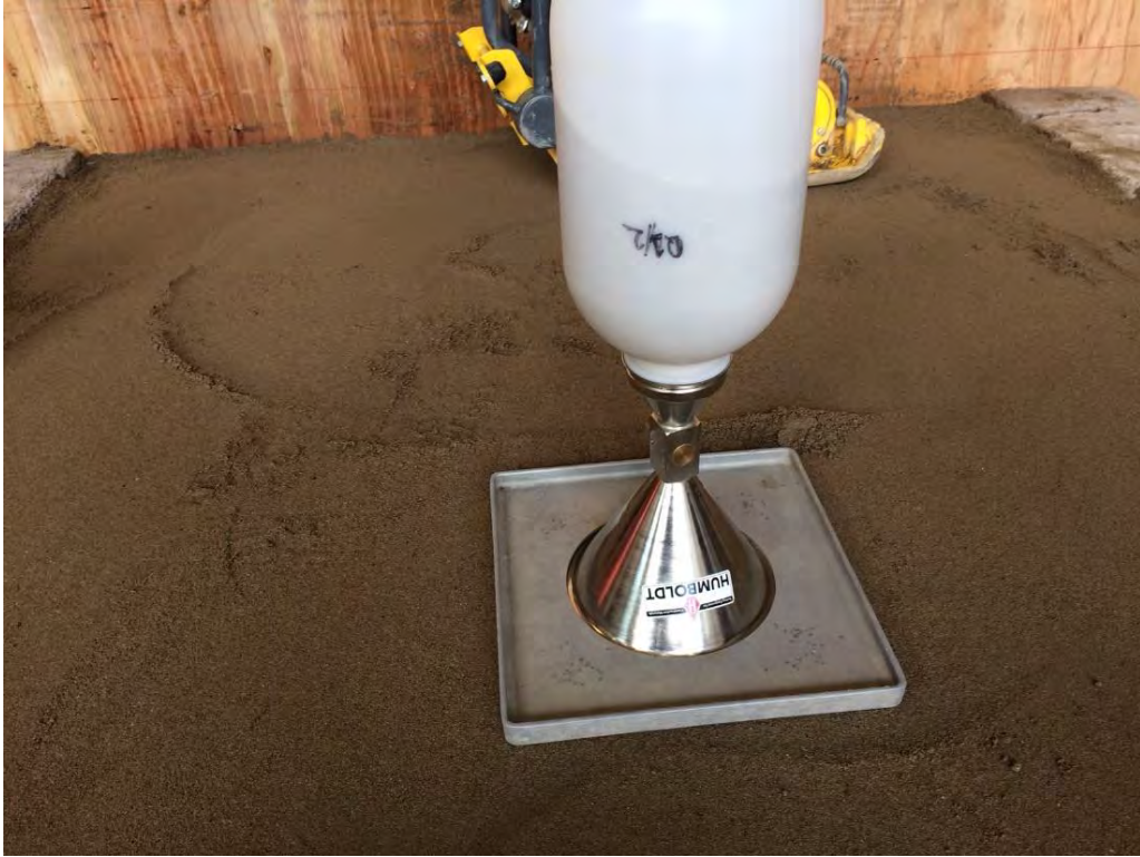
Figure A2.11 Sand cone test to measure compaction density.
