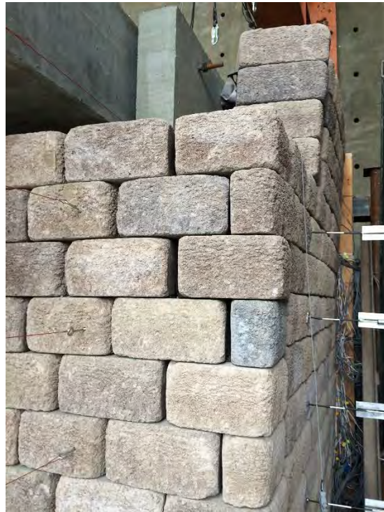
Figure A2.44 Gaps between the top corner blocks after the Northridge motion for Test 4.
