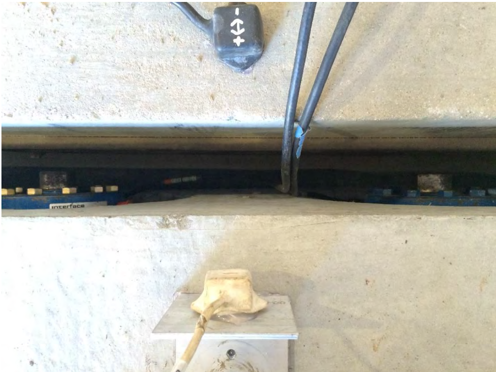
Figure A2.20 Load cells embedded at the end of bridge beam.
