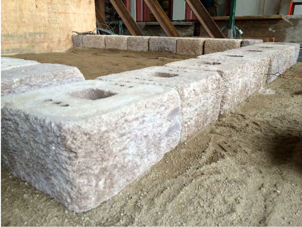
Figure A2.3 Level of the first course of facing blocks (with 1 inch elevation offset).
