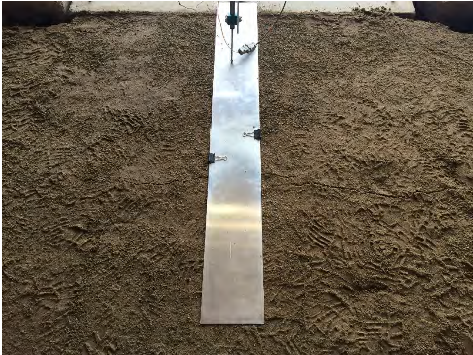
Figure A2.36 Minor crack after the Northridge motion for Test 2.
