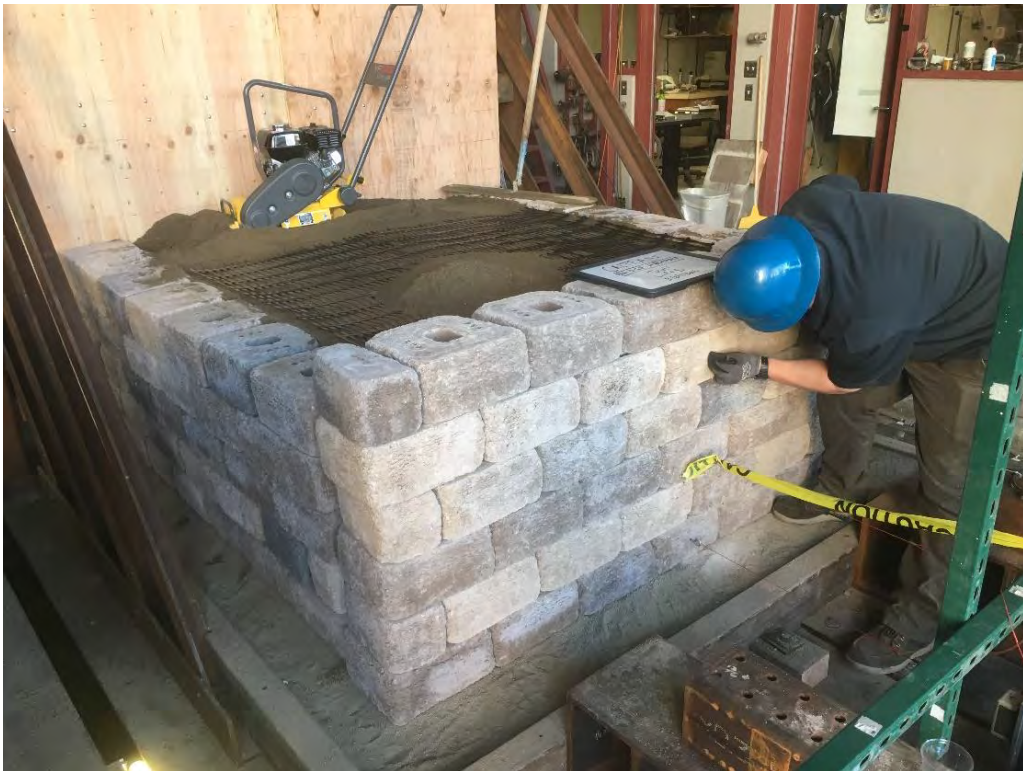
Figure A2.10 String potentiometer connected during construction.
