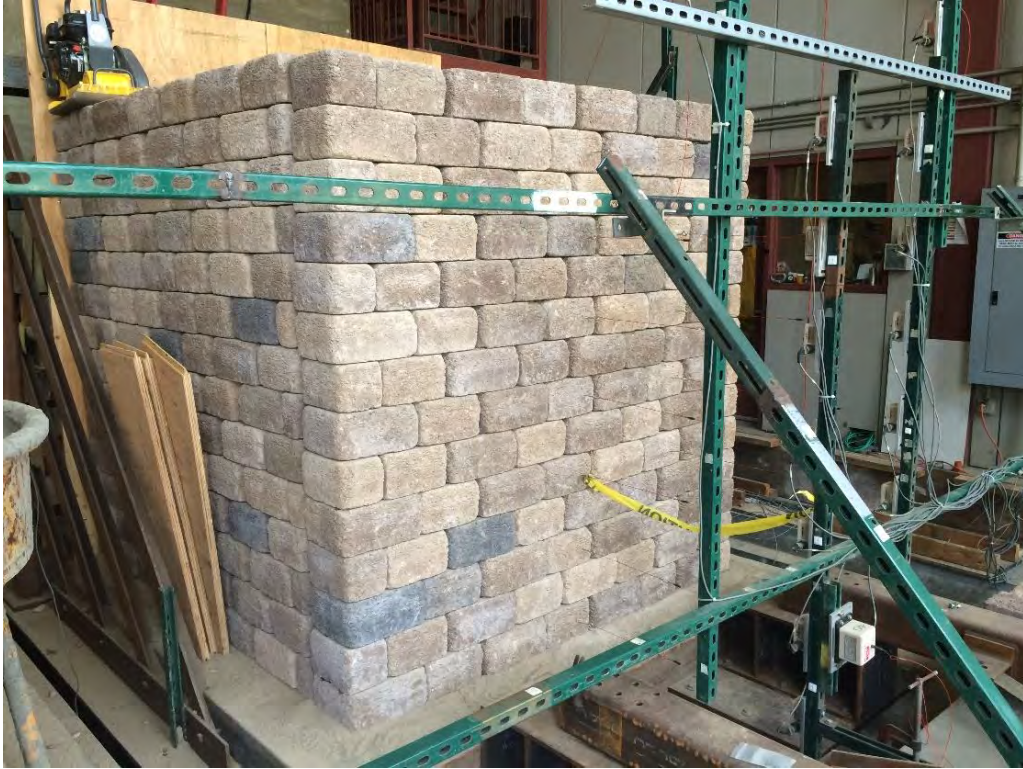
Figure A2.13 End of construction of the lower wall.
