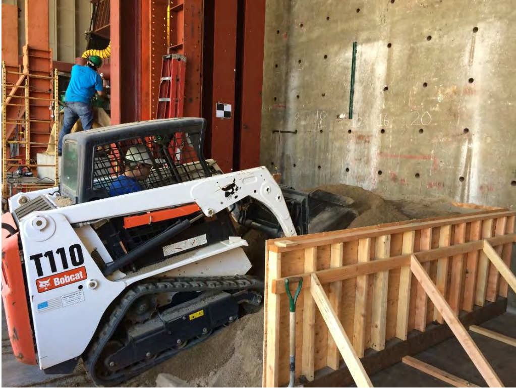
Figure A2.7 Bobcat to load sand.
