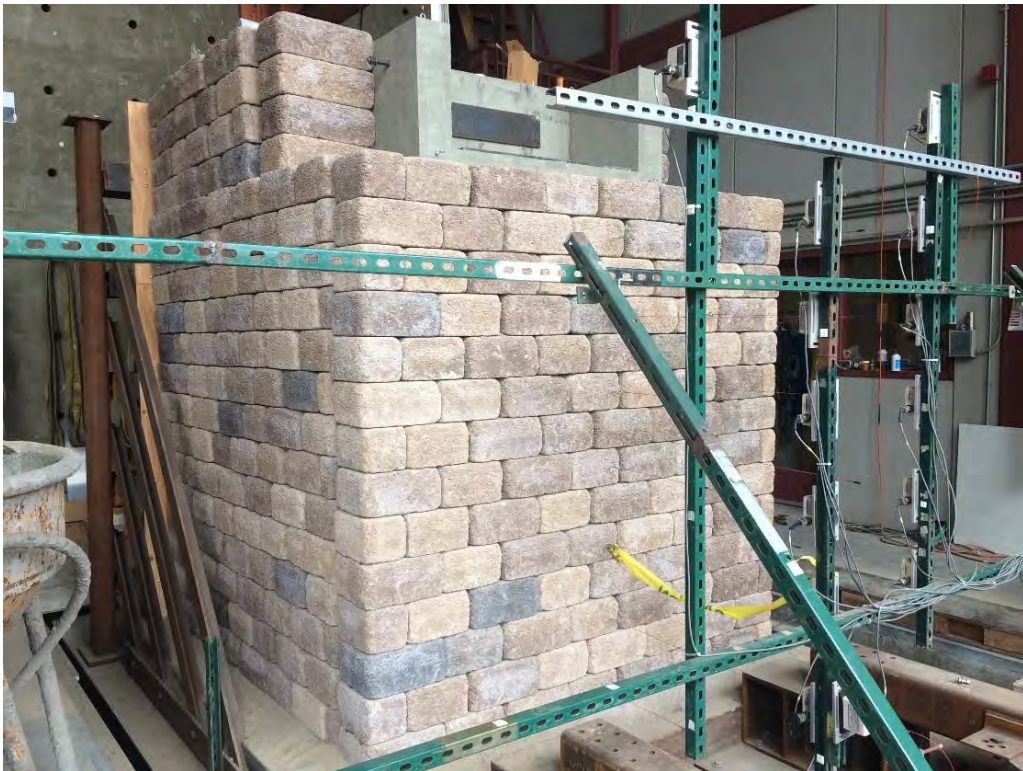
Figure A2.14 End of construction of the MSE abutment.
