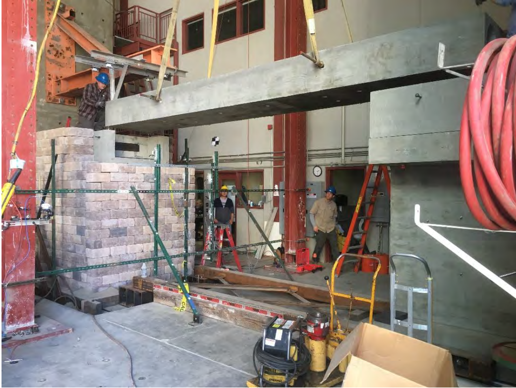
Figure A2.17 Placement of the bridge beam.
