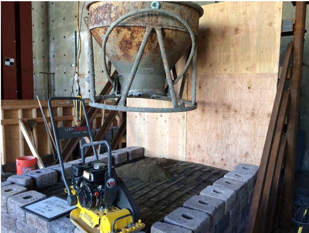
Figure A2.8 Concrete hopper to dump sand.
