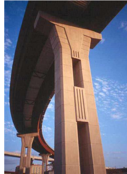
Figure 1. Typical STTG Bridge.
