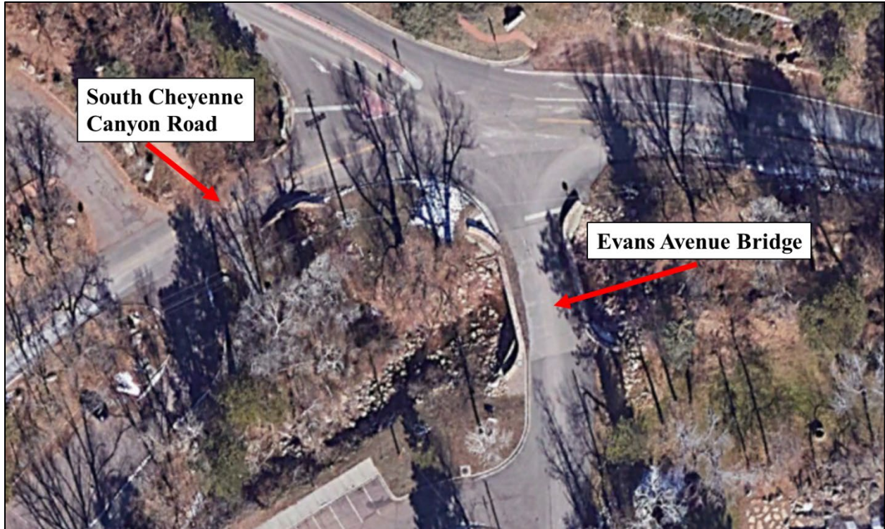
Figure 2.3 Aerial Image of Evans Avenue and South Cheyenne Canyon Road Bridges (Background Imagery from Google)
