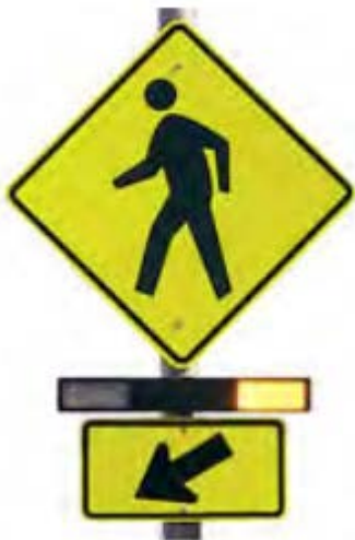
Rectangular rapid flashing beacon (Michigan Department of Transportation 2014a)
