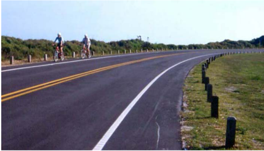
Wide paved shoulder (North Carolina Department of Transportation n.d.)
