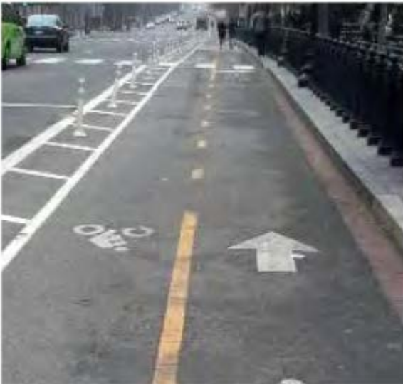
Separated bike lane (or cycle track) (Michigan Department of Transportation 2014a)
