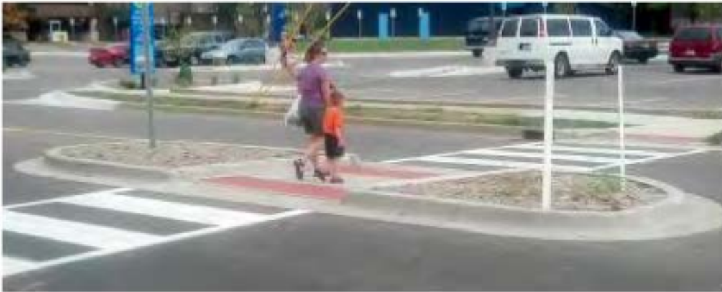
Pedestrian refuge island (Michigan Department of Transportation 2014a)
