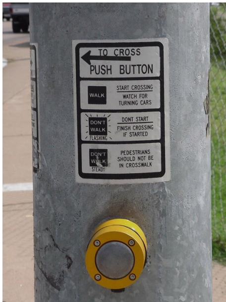
Traffic signal with pedestrian push button (Burden 2006b)
