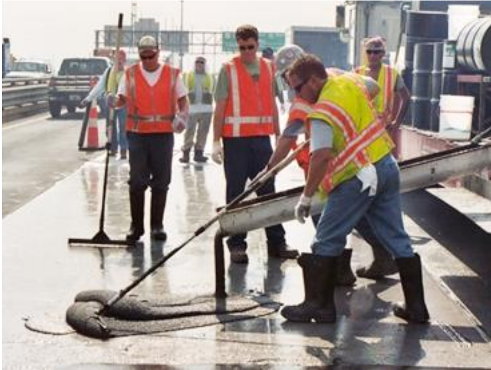
Figure 2.2. Typical placement of slurry concrete overlay (Courtesy: Transpo)
