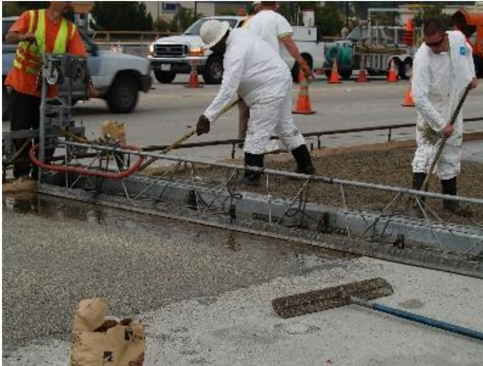
Figure 2.3. Typical placement of premixed polyester concrete overlay using a vibratory screed (Courtesy: KwikBond Polymers).
