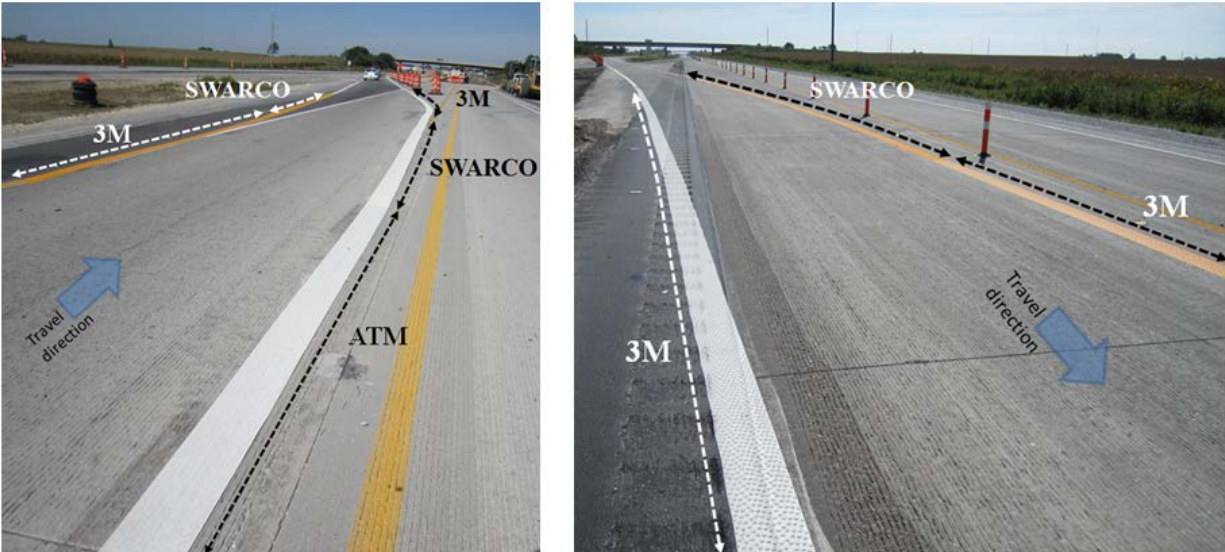
Figure 8. Tape products within the leading (left) and trailing (right) sides of the crossover
