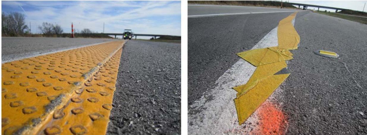
Figure 13. End of project condition for yellow edge lines leading into the crossover
