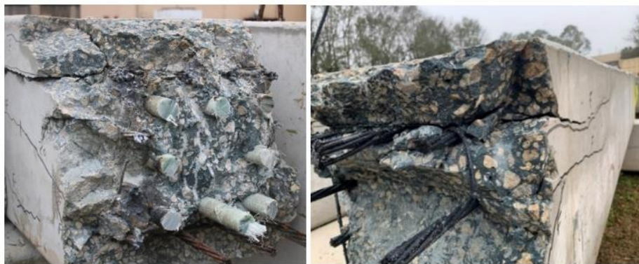
Figure 127: Two examples of the splitting cracks
