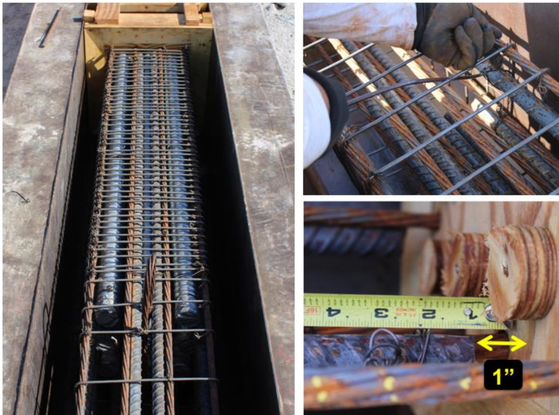
Figure 51: The spirals, strands and bars configuration
