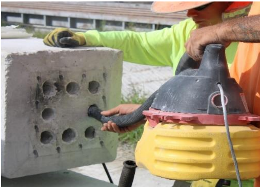
Figure 58: Drilling (top) and cleaning (bottom) the holes for unforeseen splice specimens
