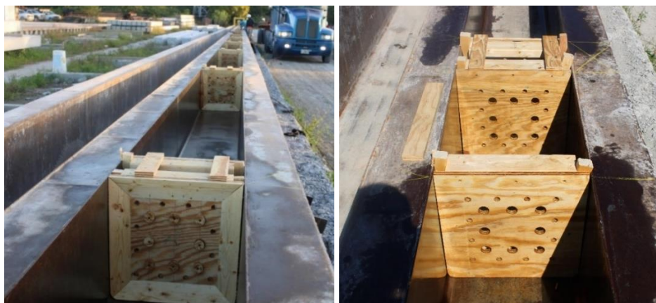
Figure 46: Wooden headers arrangement in casting bed
