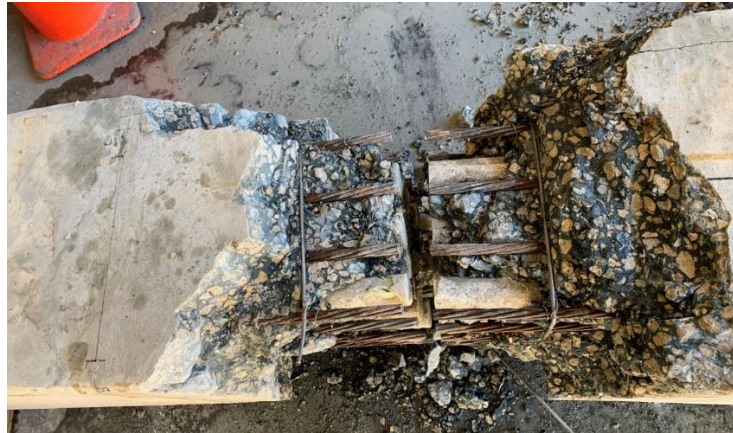
Figure 72: A photo of the Specimen 1 after test
